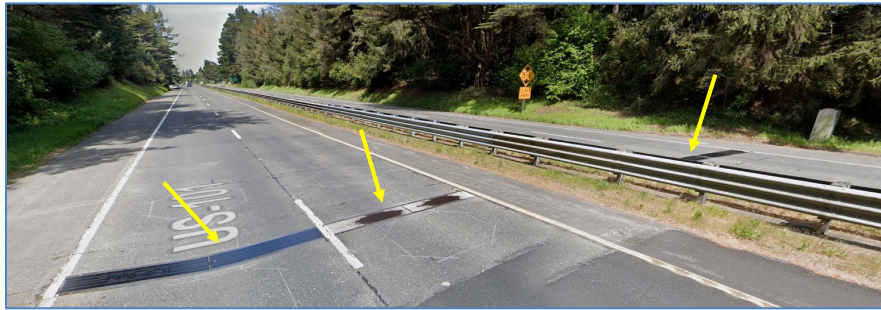
Figure 4-6: Weigh-in-Motion Station at Loleta on US-101
