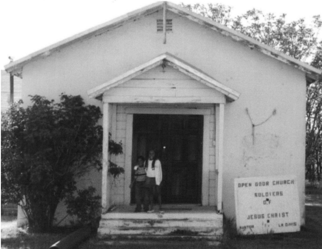
Figure 49: The doors of the Open Door Church, in Fairmead, are now closed, and the building is slated for demolition to make way for the expansion of the county dump (courtesy of the Brown family).
