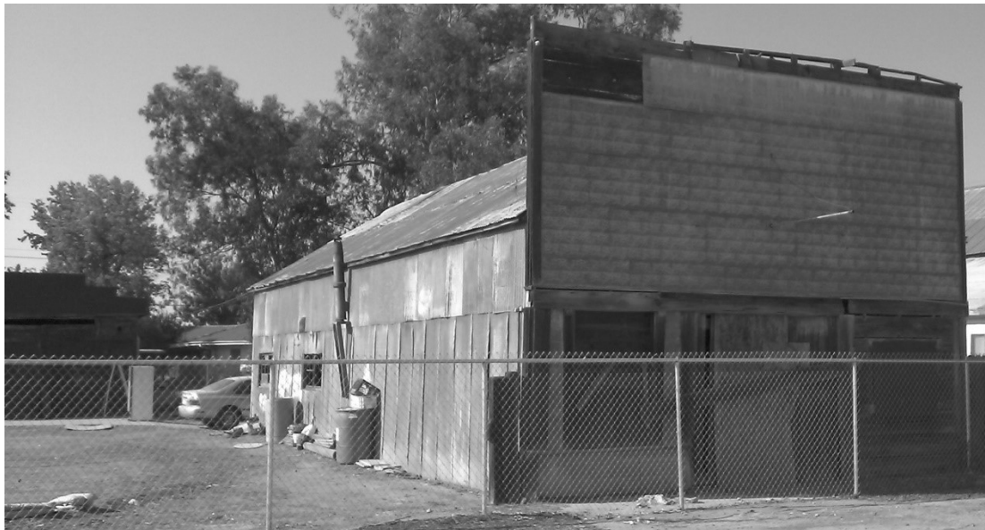
Figure 33: One of two structures in Bowles (formerly Bowles Colony) that appear to have originally been used as businesses (contemporary photo by author).
