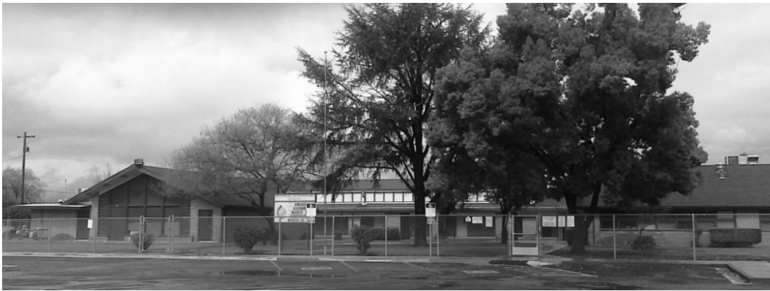
Figure 59: The current Fairmead Elementary School is used by fifth graders from Chowchilla and Fairmead (Photo by author).
