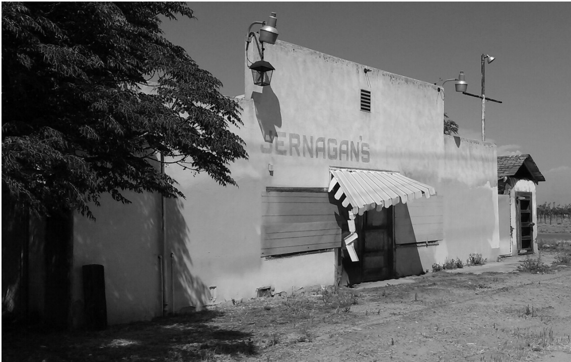
Figure 102: Shell of Jernagan's store in Teviston. In 1959, Teviston first received water service from a tap near this store. This photograph was taken on my first visit to Teviston, in 2015, where we were accompanied by Benny Beavers and C. J. Jones as we located (contemporary photo by author).
