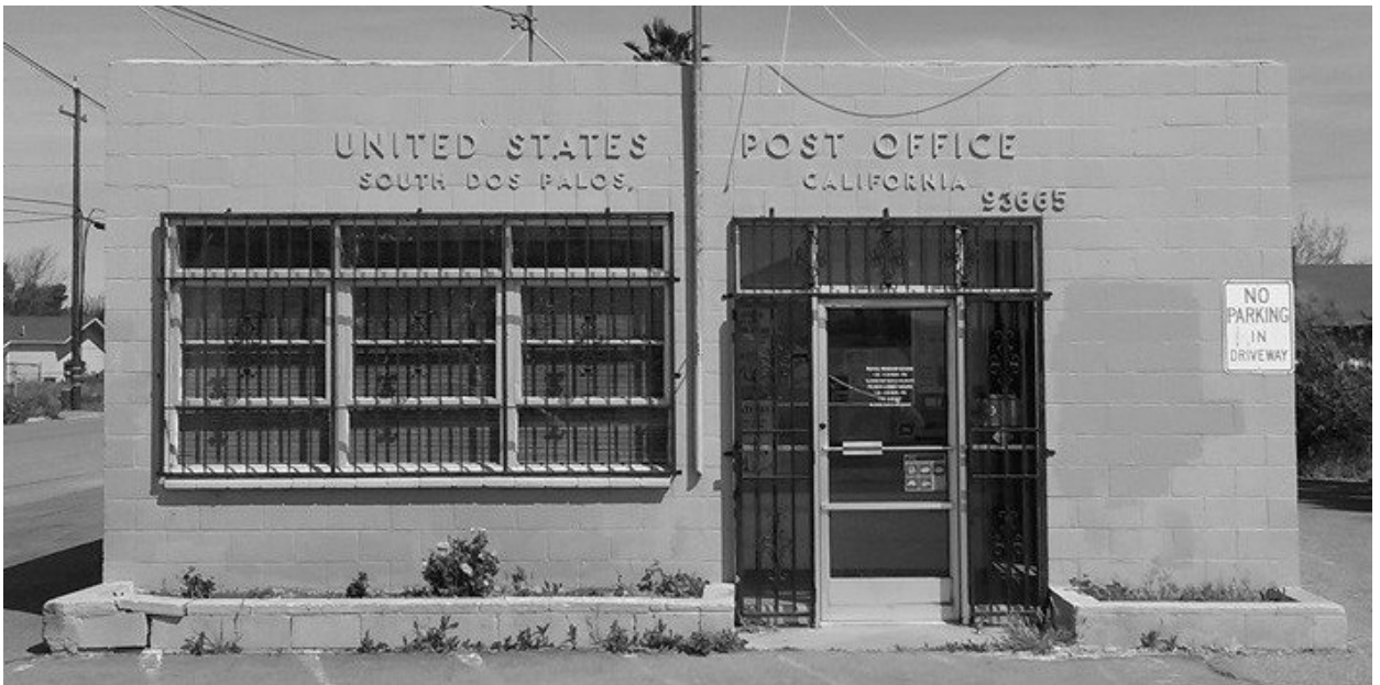
Figure 92 South Dos Palos Post Office (contemporary photo by author).
