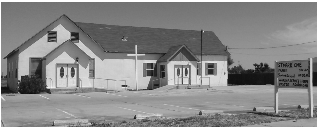
Figure 55: St Mark CME Church in South Dos Palos (contemporary photo by author).
