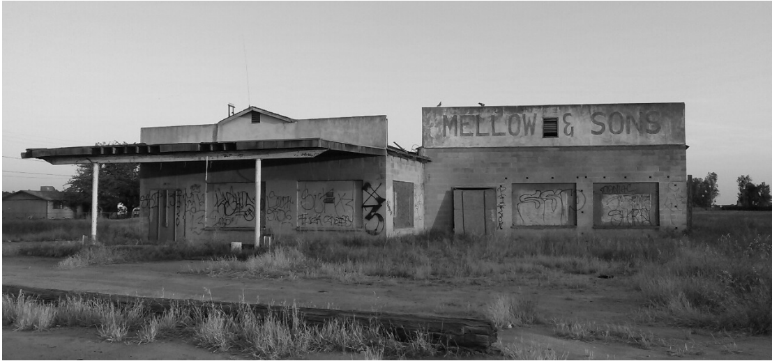
Figure 41: Mellow & Son's Wrecking Yard, in Teviston (contemporary photo by author).
