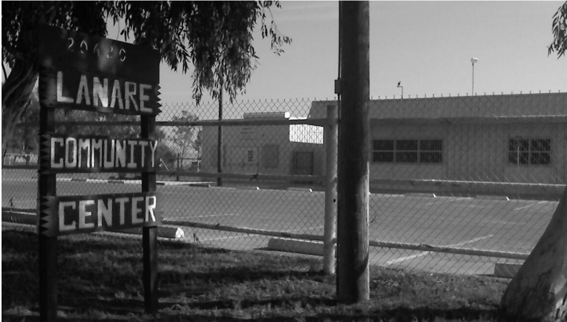
Figure 64: The Lanare Community Center (contemporary photo by author).
