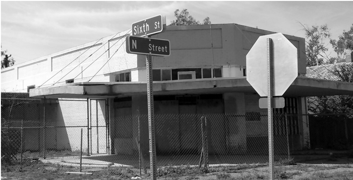
Figure 19: Boarded up storefront in South Dos Palos (contemporary photo by author).
