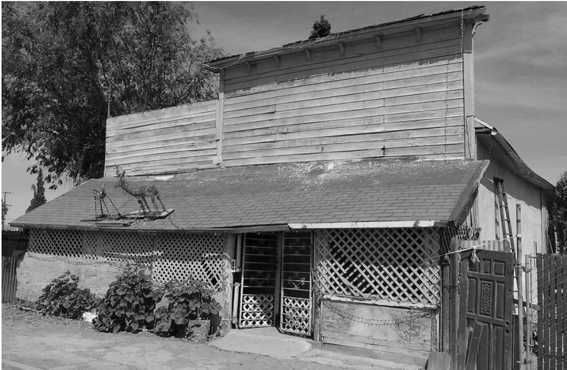
Figure 42: Converted commercial building in South Dos Palos (now a residence). Referred to as the "candy store" by informants who fondly remembered the penny candy counter from their childhoods (contemporary photo by author).
