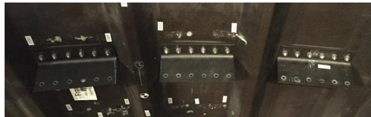
(b) C-frame only removed (shear ties mounted)
