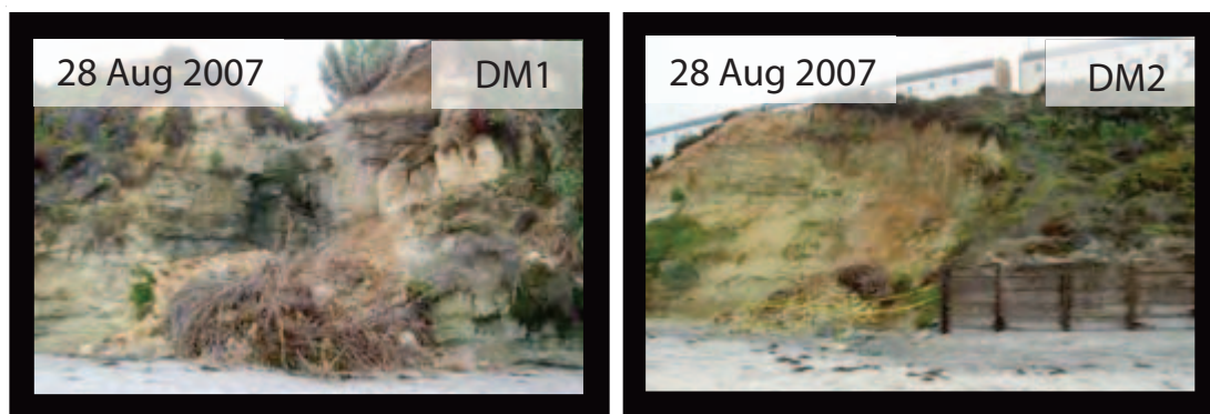
Figure 5-11: Photographs of cliff failures surveyed using Terrestrial Laser Scanning in Del Mar.
