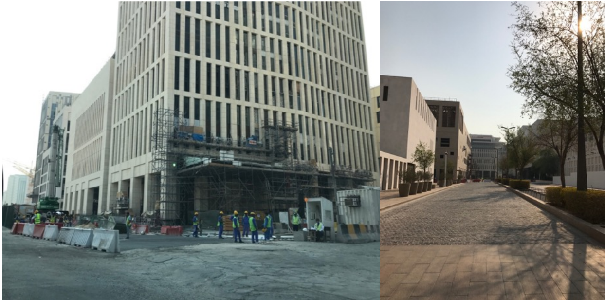
Figure 9.1: Msheireb Project Site Doha, July 2017.
