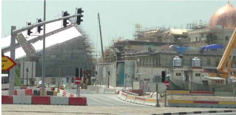
Figure 6.9: Katara Plaza Construction Doha, May 2016 Photo: Riem El-Zoghbi
