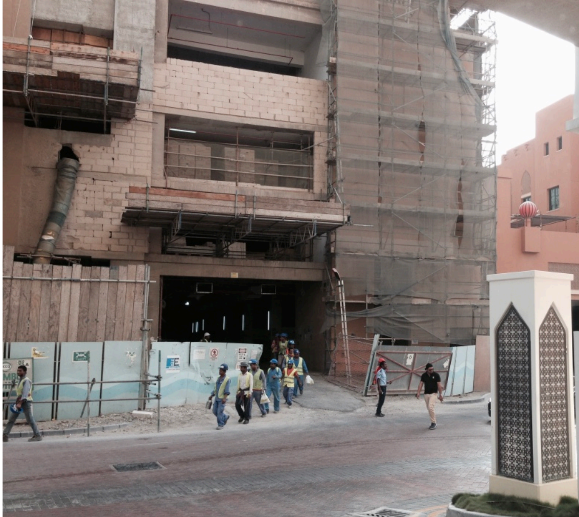
Figure 7.7: End of Worker Shift, The Pearl Porto Arabia, Tower 29 Doha, May 2016
