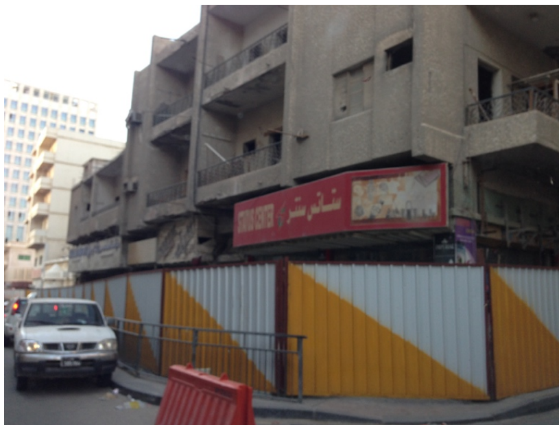
Figure 9.2: Typical Building Slated for Demolition Doha, April 2016.
