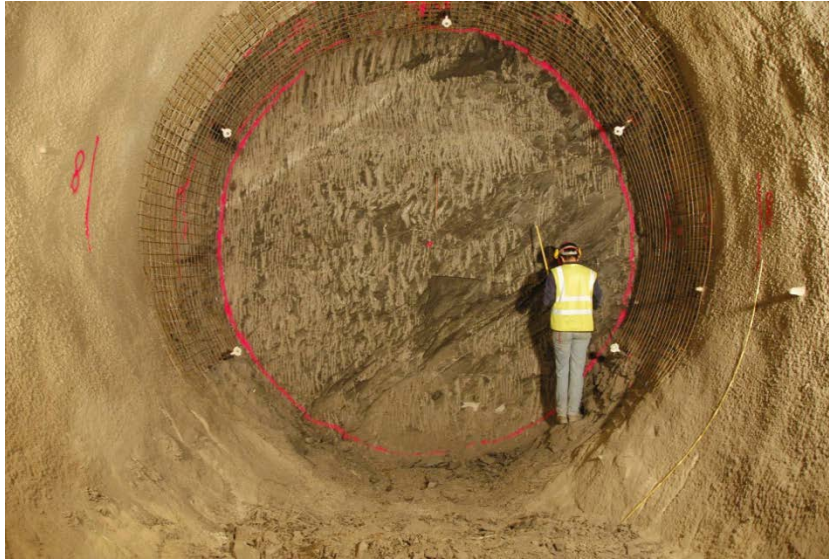
Figure 4.38. View of FE tunnel face from the FE niche showing beddings dipping 45^\circ (Vietor, 2012).
