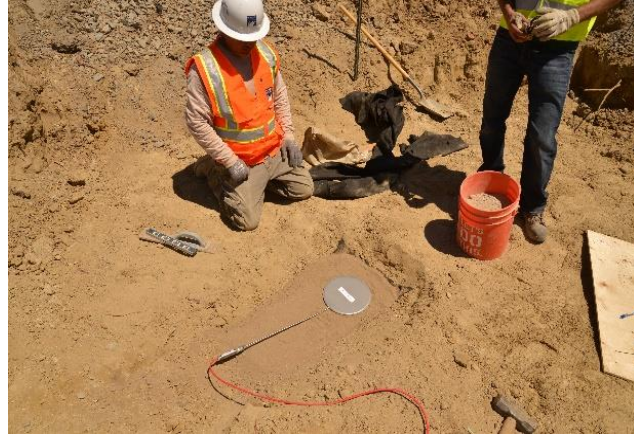
b) Installation of pressure cell
