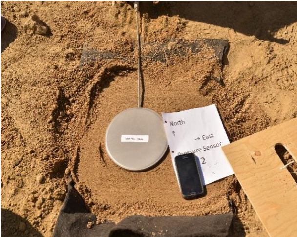
a) Installing pressure cell with directions
