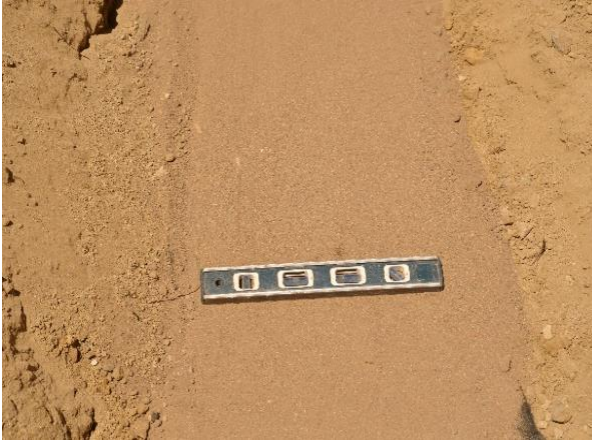
a) Leveling of subgrade
