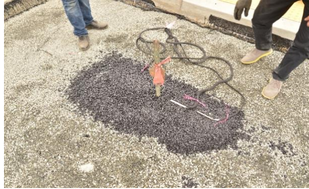
b) Placing strain gages on asphalt
