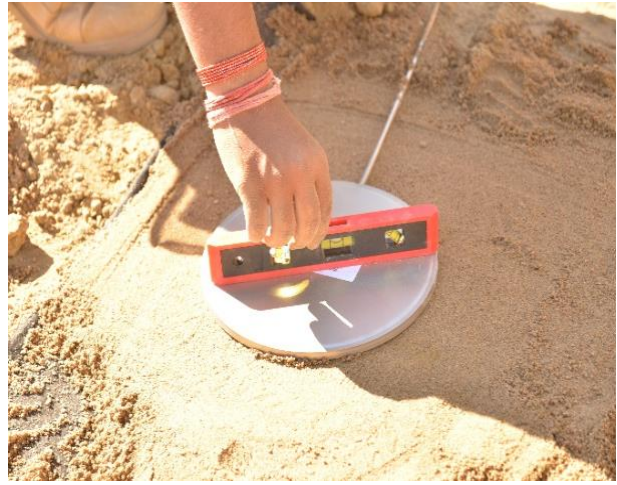
b) Leveling of pressure cell
