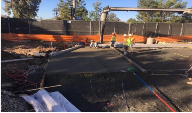
a) Permeable concrete placement
