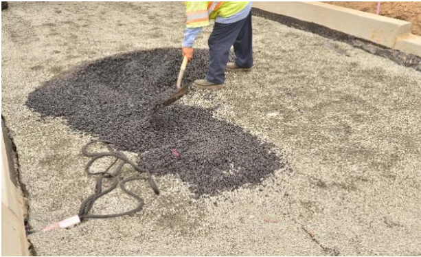
c) Pouring of HMA on strain gages
