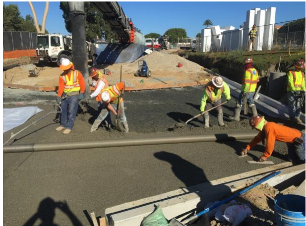
d) Compaction using hand floats
