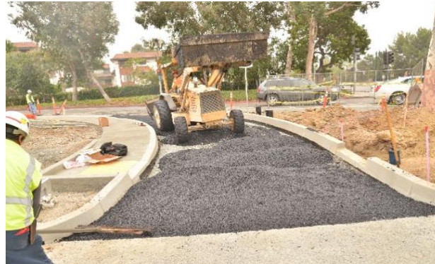
d) Pouring of HMA on test section
