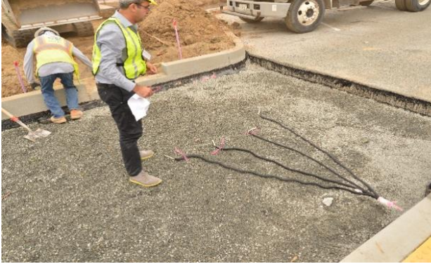
a) Placing strain gages
