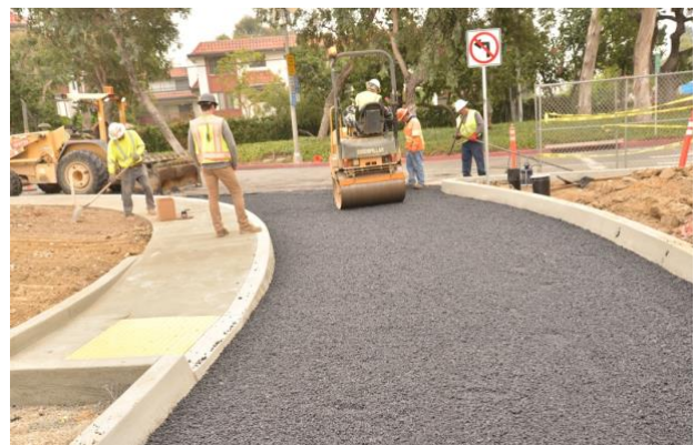
b) Compaction using static roller
