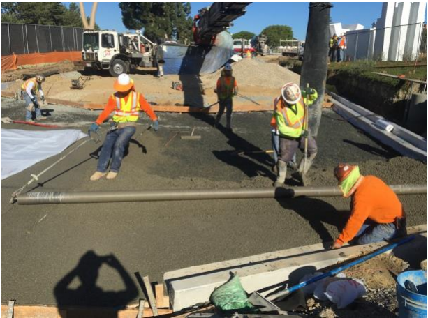
c) Compacting concrete using roller screed
