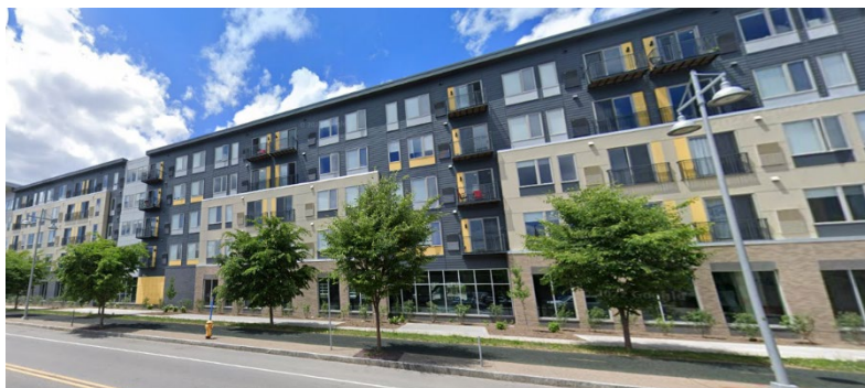
Figure 8. New Development on Union Street (the "wall"); Image from Google Earth.
