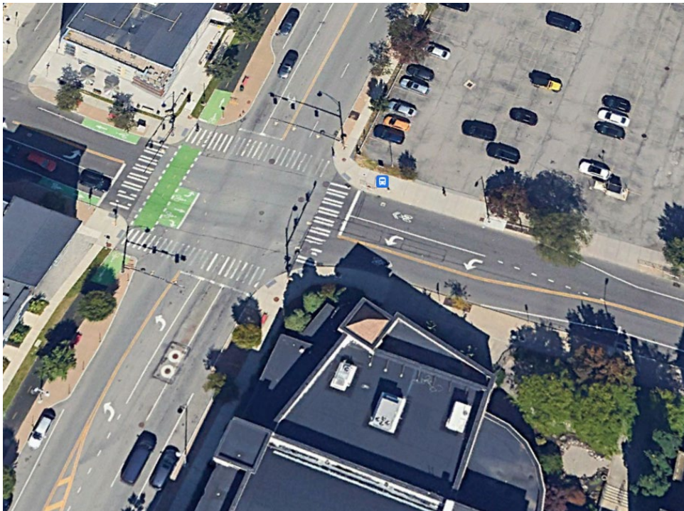
Figure 14. Turning Lane at Union Street and East Avenue (Google Earth, 8/2023).
