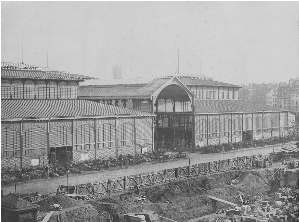
Figure 2. The Les Halles pavilions, photographed in the 1860s during their construction by Charles Marville. Courtesy of the Prints and Photographs Division of the Library of Congress, Washington D.C.
