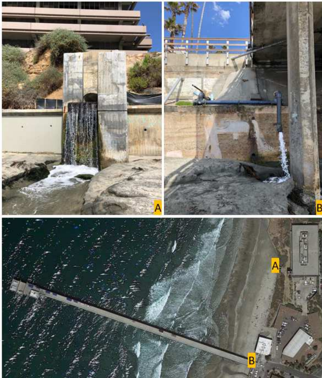
Figure 9: The two main wastewater outfalls, and their locations on the beach. (A) The outfall serving Birch Aquarium, Hubbs Hall, and NOAA-SWFSC. (B) The outfall serving Kaplan Aquarium and holding tanks.
