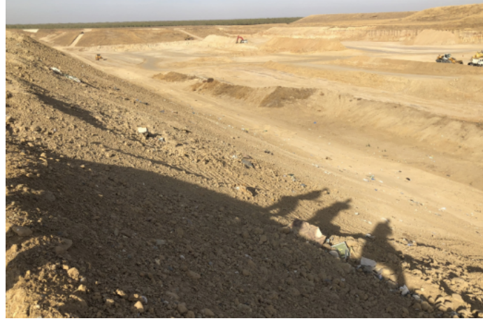
Figure 3.25: At the MCRWM site a new cell is being developed, such that, the bank shown in the image has no membrane and only a dirt cover.
