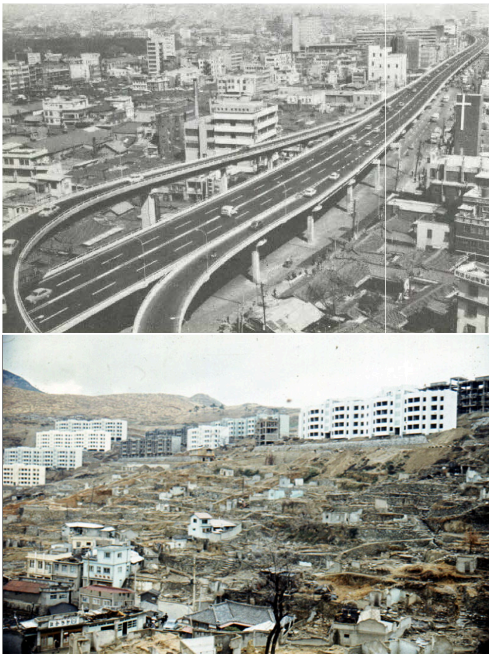
Figure 3-6. Urban renewal programs, from Sam'il Expressway (above) and public housing/slum clearance project (below), took place during Mayor Kim's five-year tenure. (Image source: H. Kim 1969; The National Archives of Korea)
