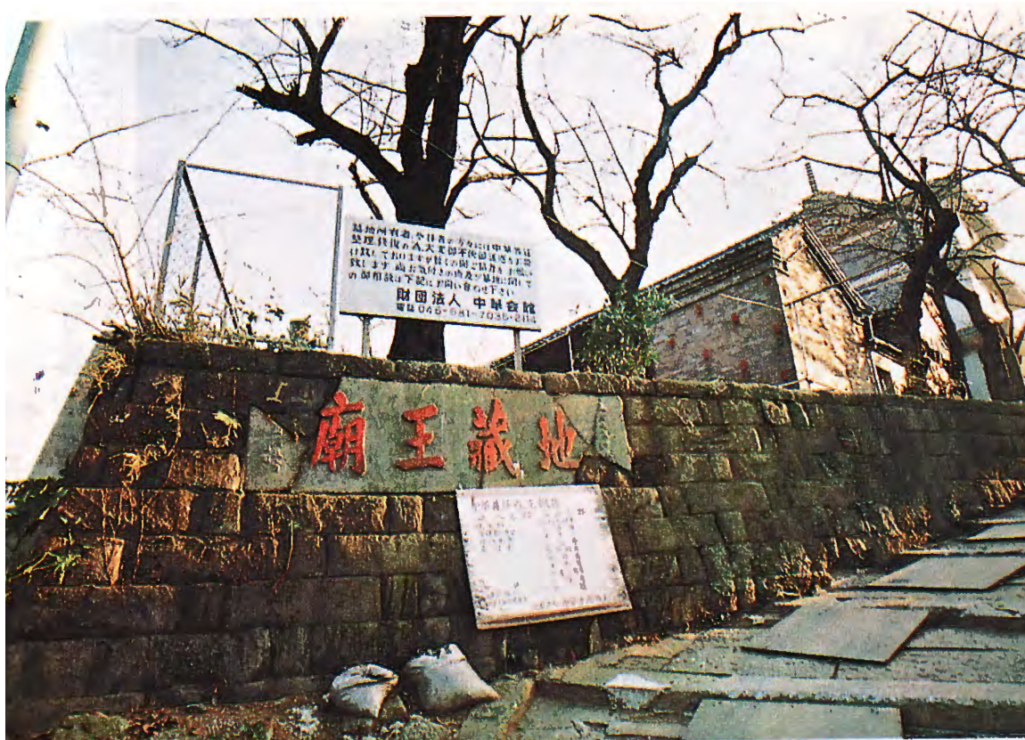
Figure 2-12. The entrance to the Chinese cemetery before its restoration in the early 1990s. (Image Source: Hengbin huaqiaozhi, 1995)
