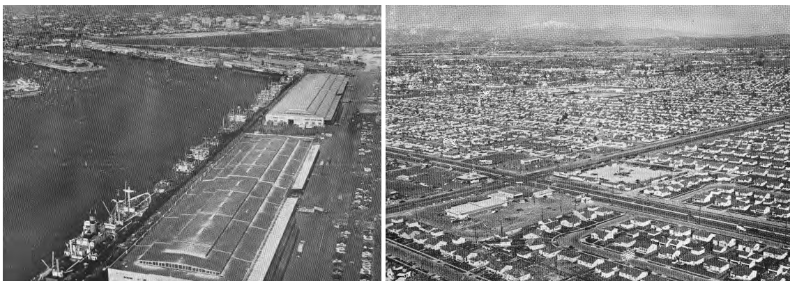
Figure 2-5. The Japanese delegates took an inspection tour of harbor facilities in Long Beach (left) and housing tracts in Portland (right). (Source: Hiranuma 1954)
