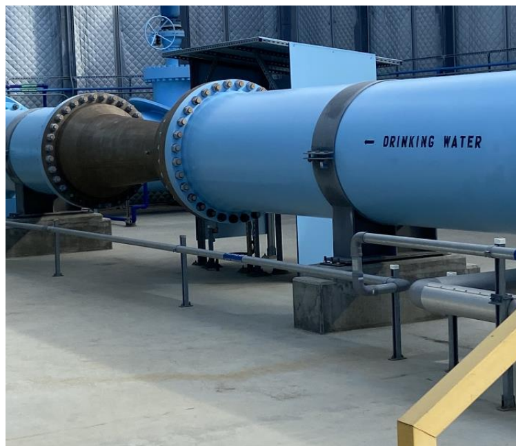
Figure 9.1 Point of delivery for the Carlsbad Desalination Facility. Each contract that focused on water provision included a point of delivery, after which the entity operating the facility no longer holds responsibility over water quality and use. In the figure above, the narrow black pipe is the “point of delivery” for the Carlsbad desalination facility. By the time it reaches the black pipe, water must meet all performance standards outlined in the contract (Shadowing, 12/18/2019).
