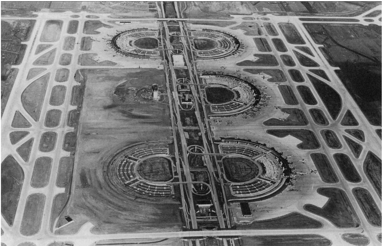
FIGURE 2.3 Gyo Obata, D/FW Airport, final terminal layout design under construction in 1973
