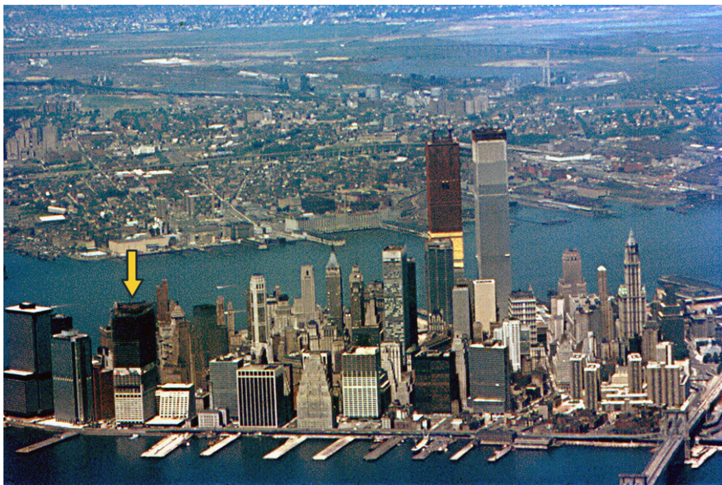
FIGURE 3.20 View of 55 Water Street (bottom left) under construction, 1971
