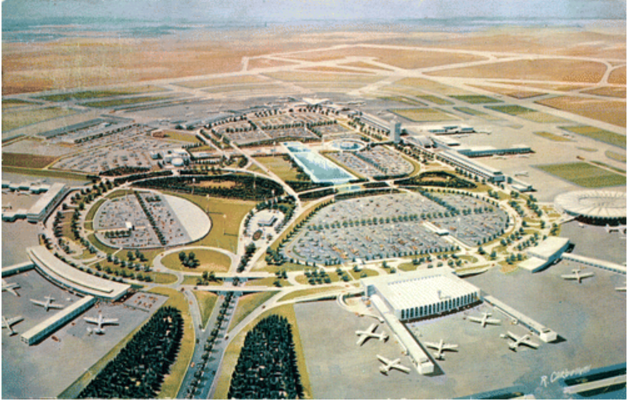
FIGURE 2.11 Terminal City plan, Idlewild, New York International Airport (now John F. Kennedy International Airport), New York. c. 1957, artist's conception of completed airport from a vintage postcard
