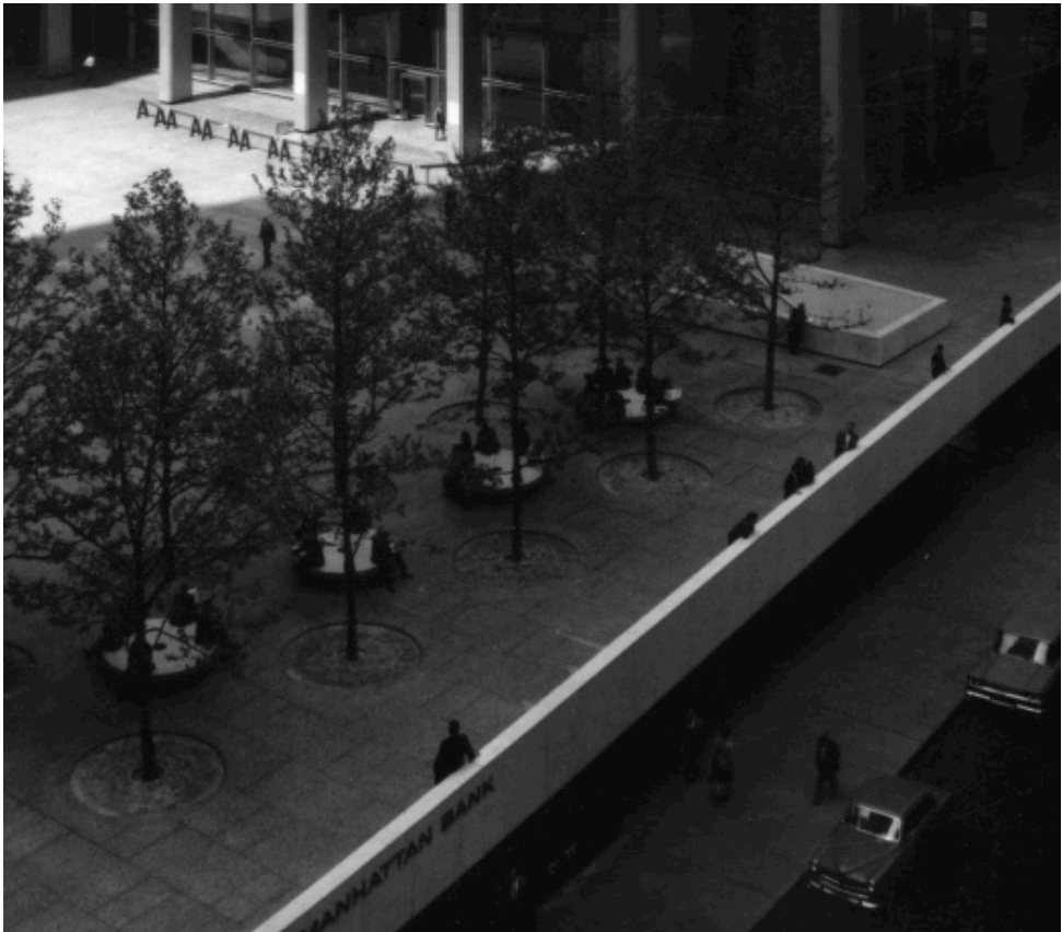
FIGURE 1.20 View of "cantilevered" section of Chase Manhattan plaza on William Street, as executed in final construction of the plaza
