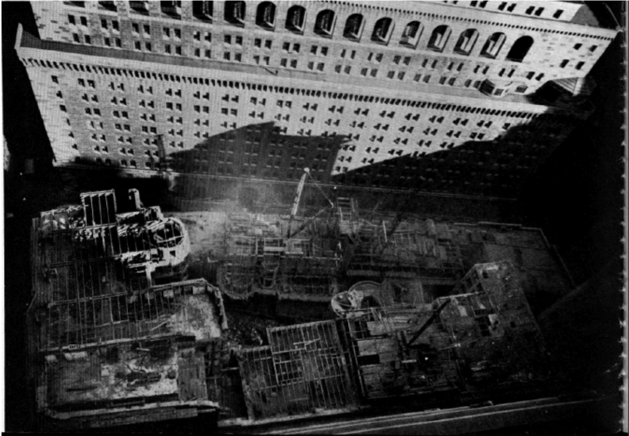
FIGURE 1.33 Demolition for future site of Chase Manhattan Bank headquarters, early 1956
