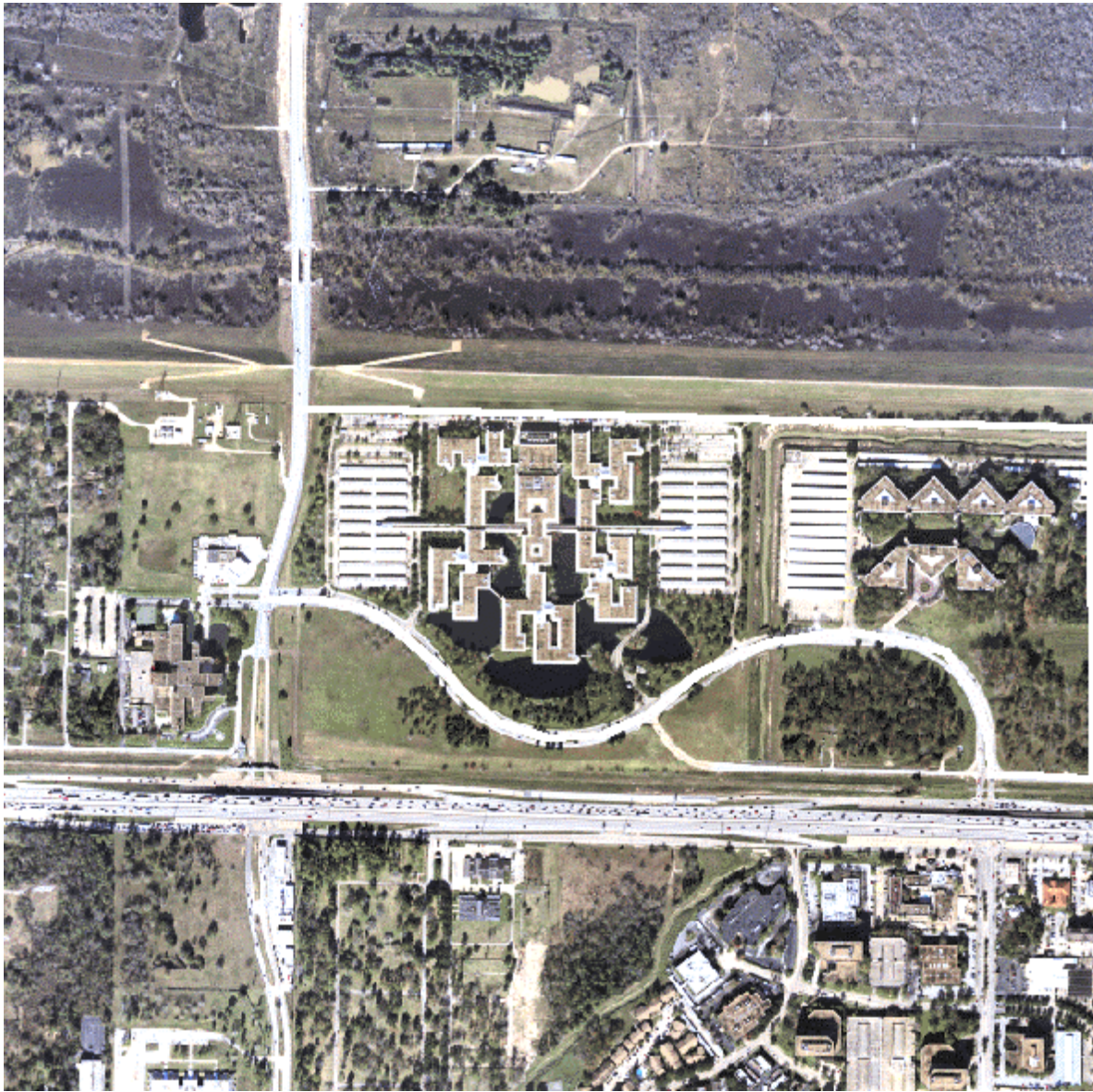
Figure 11. Aerial orthophoto of the Park Ten Place area.
