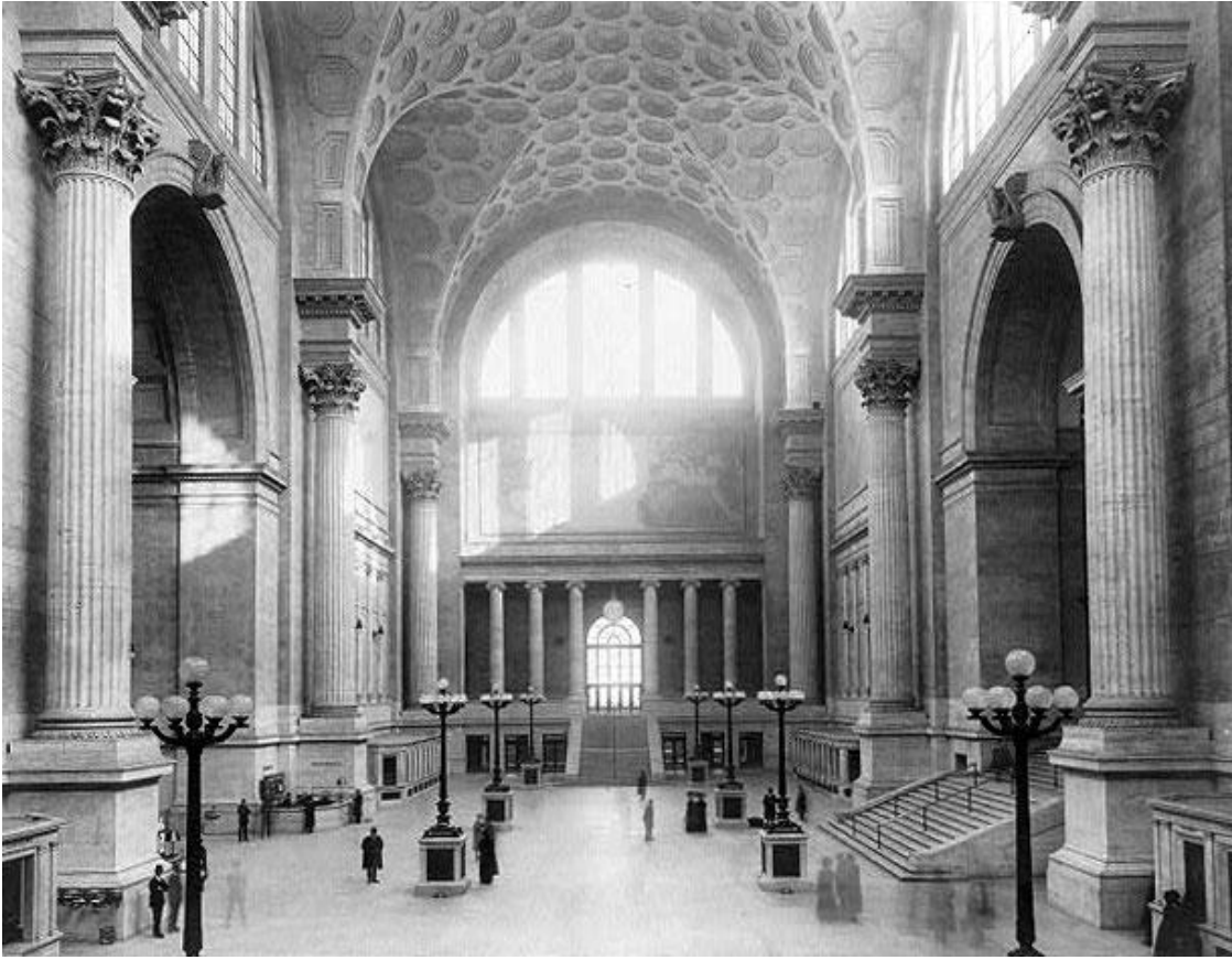
Figure 30. Main waiting room, Pennsylvania Station, ca. 1911.
