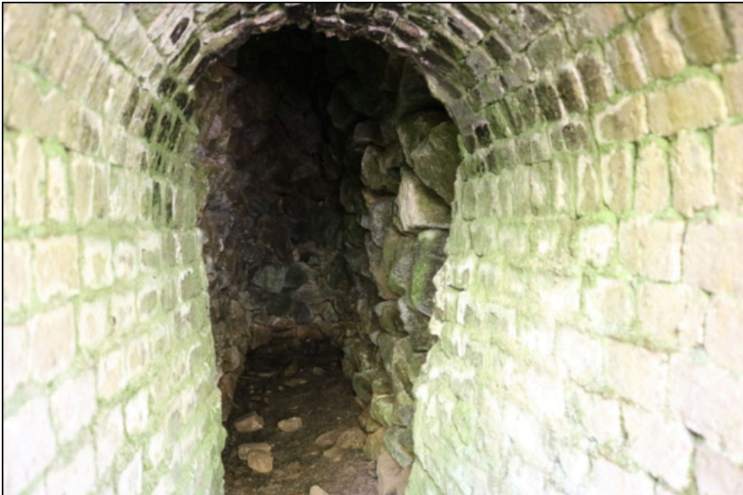
Figure 5.19 Interior fire chamber and raw lime arch, Pot 2
