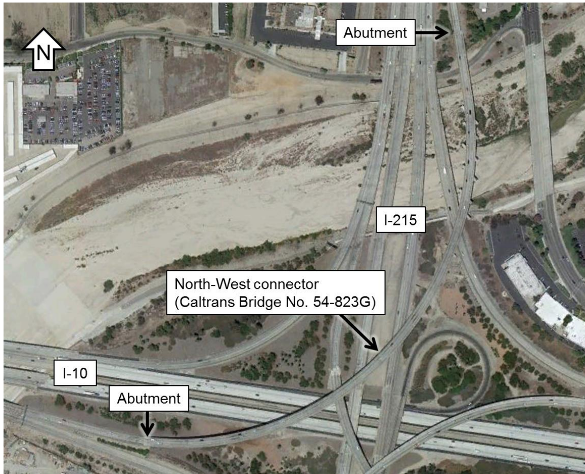
Figure 3.3: Aerial photograph of the NW connector at the I-10/215 interchange (©2013 Google - http://maps.google.com )
