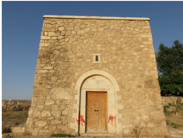
Figure 2.14. The restored church of Edremit. July 25, 2014.
