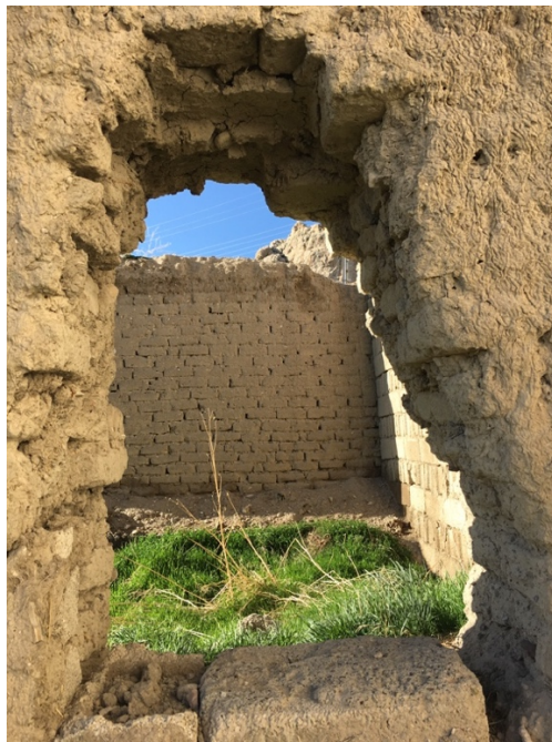
Figure 6.6. Interior of the ruined house. March 25, 2018.
