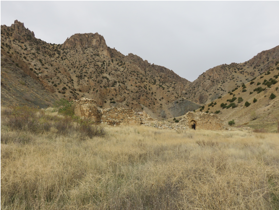
Figure 3.1. Front walls of Der Meryem monastery. November 8, 2015.
