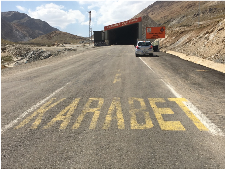
Figures 5.23 & 5.24. Entrance to the new Karapet Kar Tüneli (Karapet Snow Tunnel). August 29, 2017.
