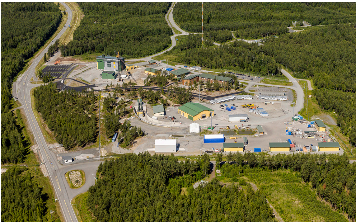
Figure 7-1. Posiva's ONKALO site in Olkiluoto in summer 2014. The ramp and entrance to the ONKALO access tunnel are visible in the center of the image. Posiva has constructed a project office and various technical buildings at the site. The infrastructure is designed so that it can be utilized for the operation of the future disposal facility.
