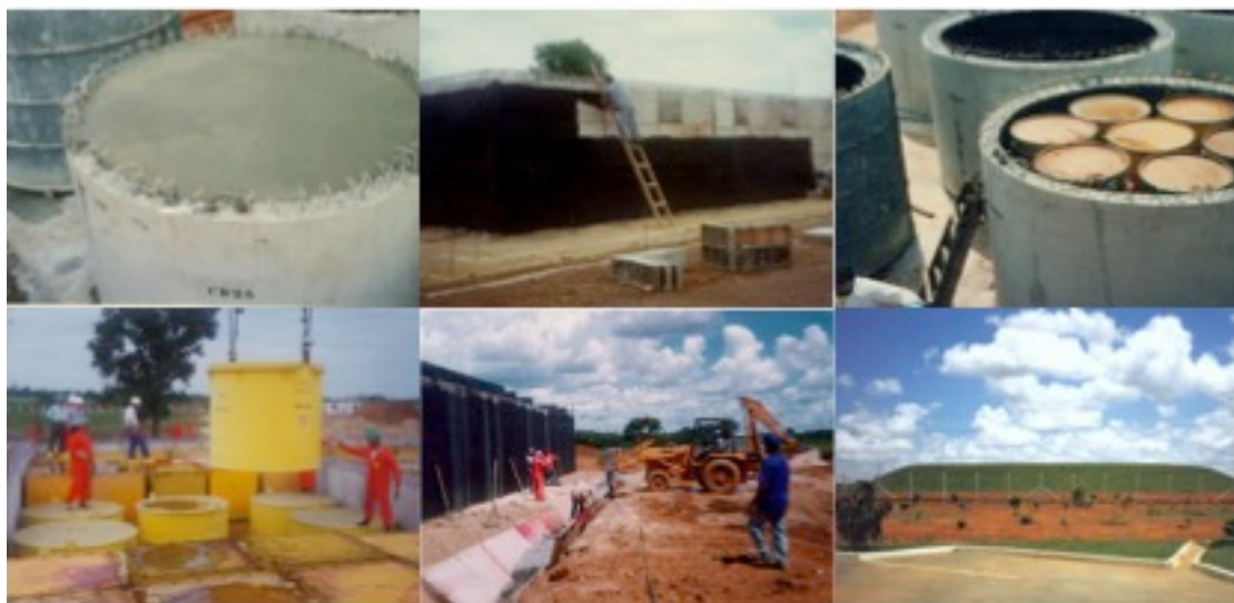
Figure 2–4. Final disposal sites in Goiânia, showing the two near-surface disposal units (vaults), and the necessary waste treatment before final disposal of packages.
