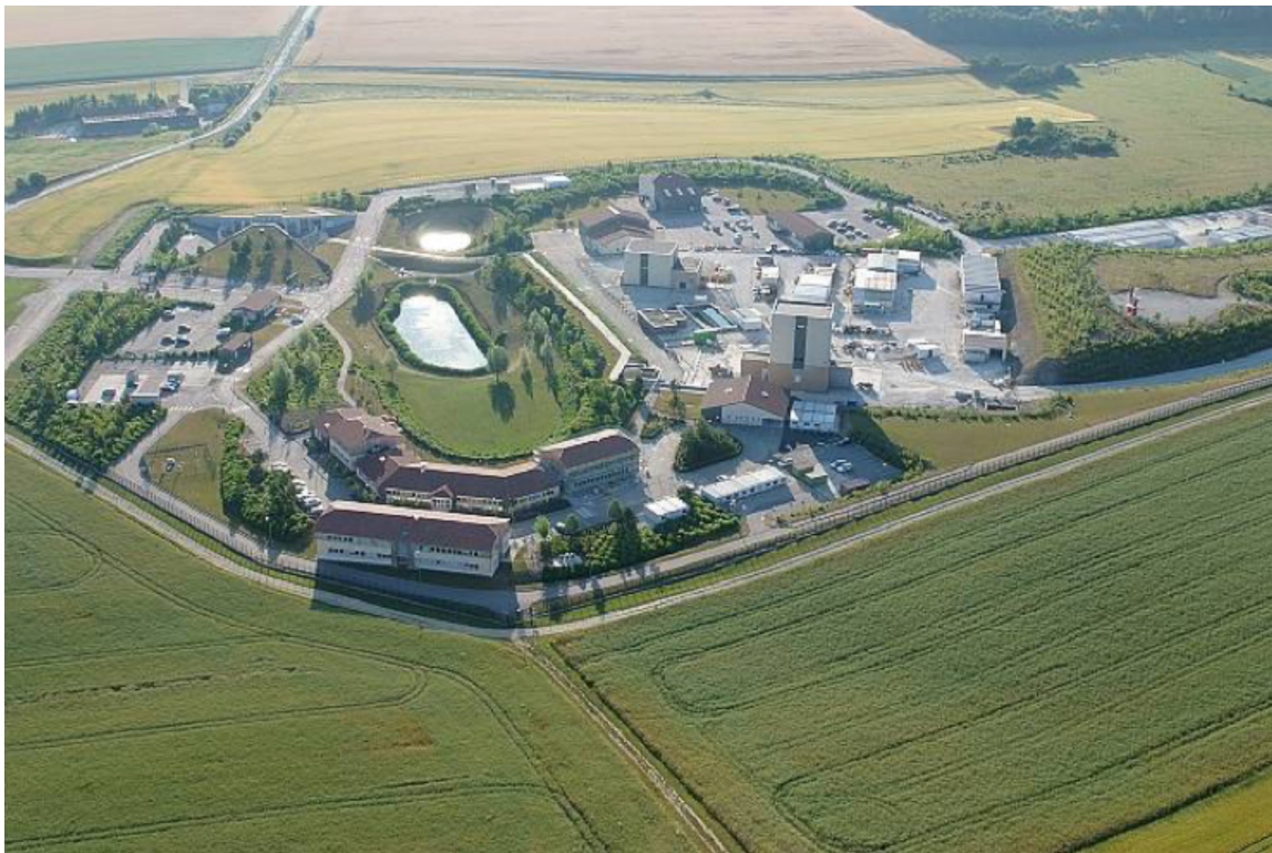
Figure 8–5. Aerial view of the Bure underground laboratory
