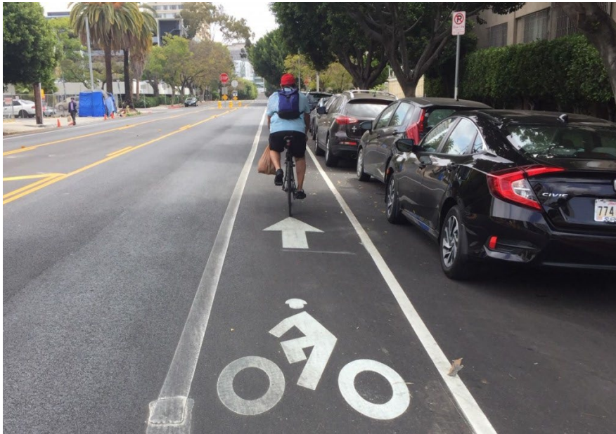
Figure 5. Constrained bike lane
