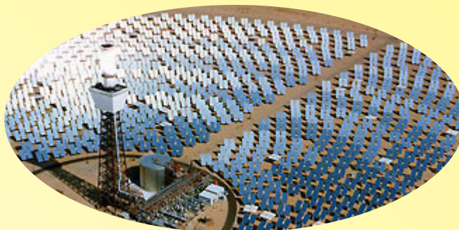
Solar Two was a proof-of-concept solar-thermal energy plant that used molten salt to capture and store the sun's heat, allowing for energy production even at night.
