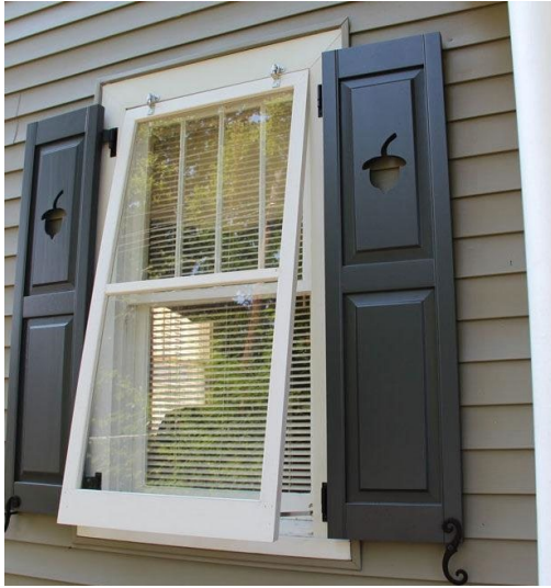
(c) Exterior storm window
