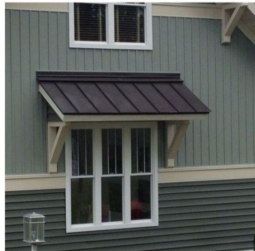
(b) Exterior overhang
