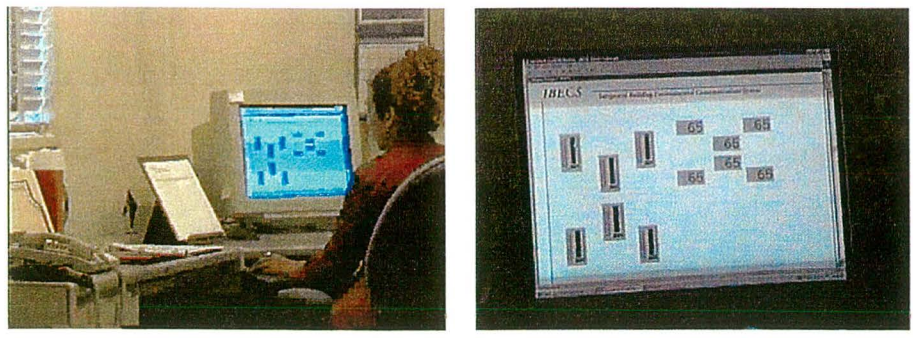
Figure 9. Left image shows occupant using IBECs to change the dim levels of the overhead lights using the computer. The right image is a closeup of the IBECs control screen. Note the six “sliders” on the left portion of the image each corresponding to a separately controlled ballast.
