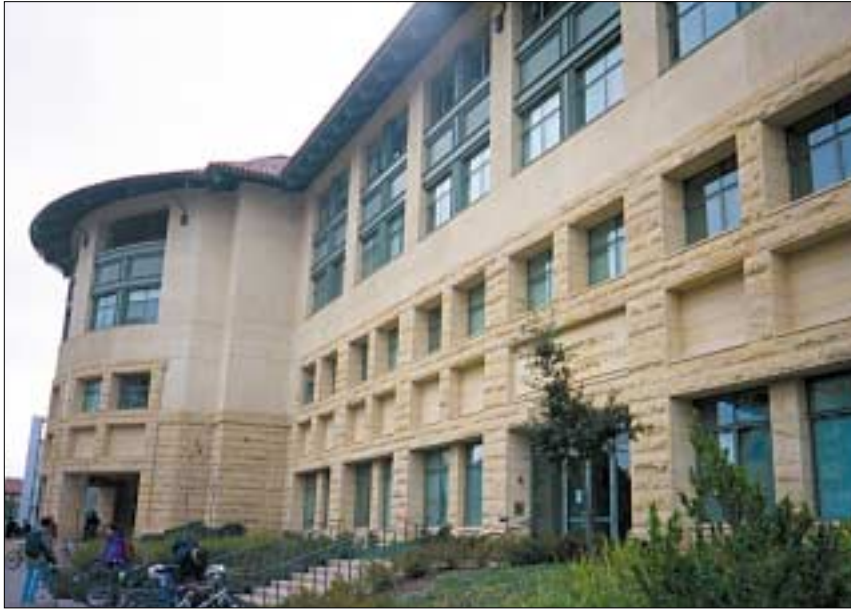
The test building in Palo Alto, CA uses a VAV system and allows individual control of thermostats. With its “changeover” system, micro-switch sensors in the windows shut off a zone VAV box if the corresponding window is open.
