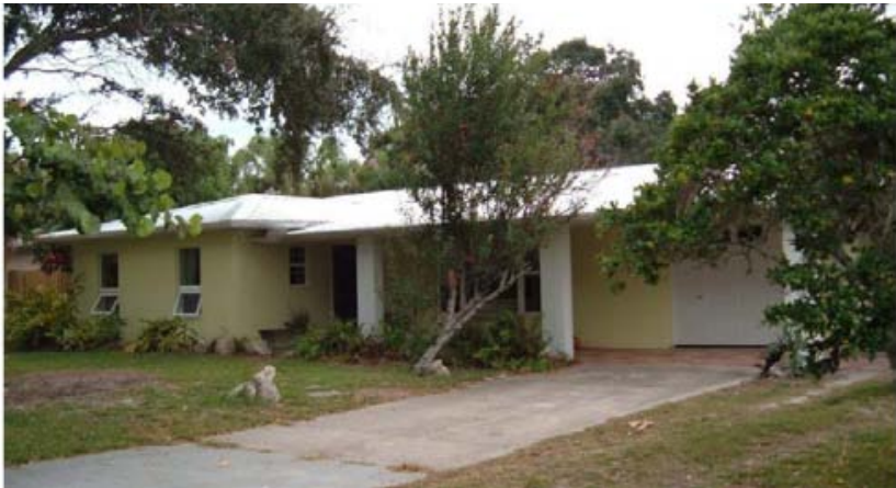
Figure 12 Phased DER home in Florida. Image courtesy of Danny Parker at the Florida Solar Energy Center.
