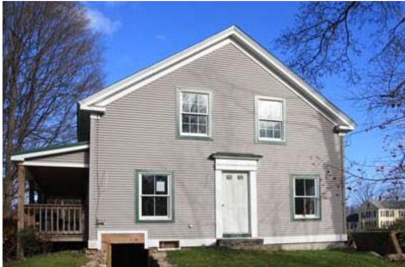
Figure 6 Front facade of the Belchertown DER. Image courtesy of the Building Science Corporation.
