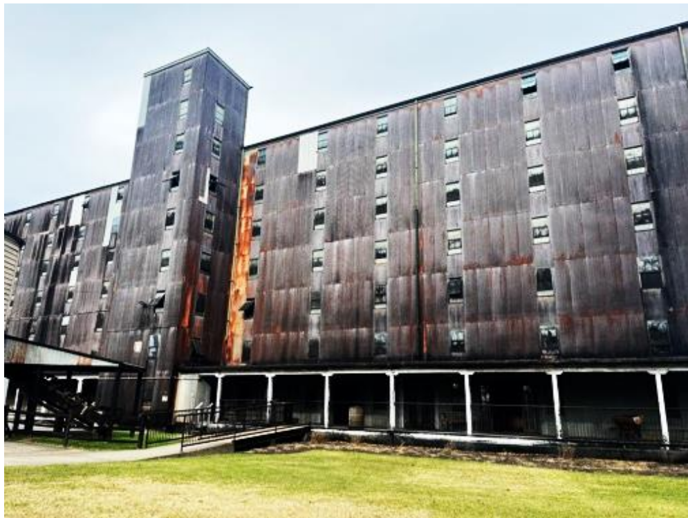
Fig. 5. Whiskey fungus grows on a bourbon aging facility in Louisville, KY. Photo: Maiza Hixson, 2023.
