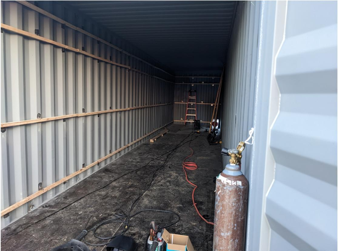
**Figure 3.4:** Image of interior of ISBU container for EcoHus construction. Steel brackets were welded on to the walls, and 2x2 lumber was secured as framing and backing for insulation and interior finishes.
