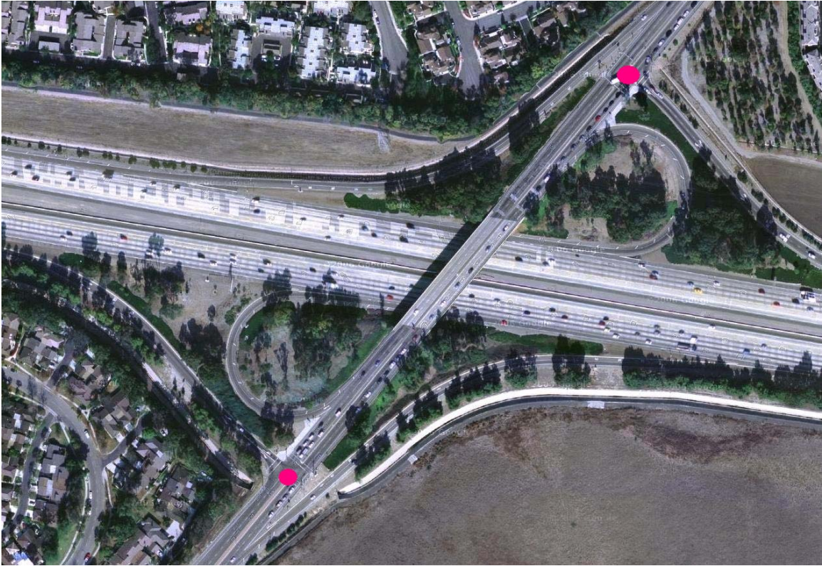
Figure 4.1 Two Caltrans controlled signals at a freeway interchange
