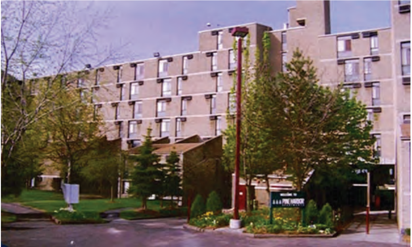
10 Seventh Street apartment building facade (Buffalo)
