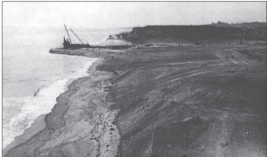
Figure 7. Photo similar to Figure 6, but looking north from Station B.
