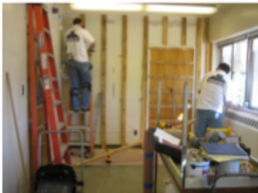
Closing off a door and adding tack board for posting and soundproofing.
