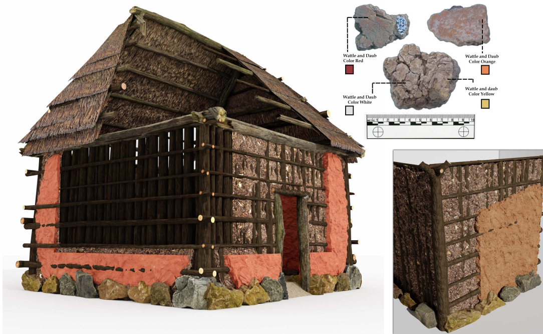
Figure 30. Wattle-and-daub located at El Ocote (Arellano G. 2014) and Hypothetical building reconstruction (M. Dueñas).
