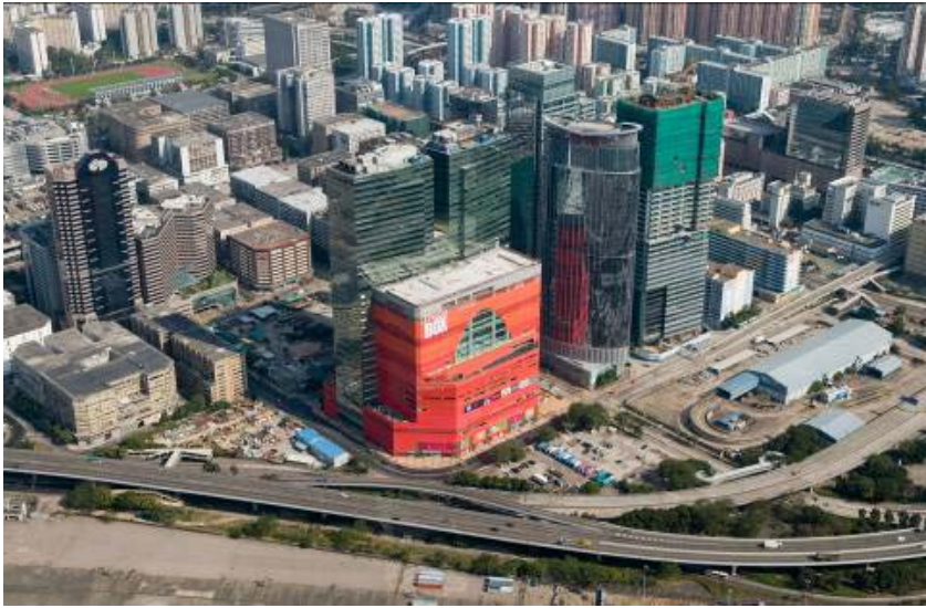
Figure 12. Aerial of the MegaBox, Source: Jerde Partnership.
