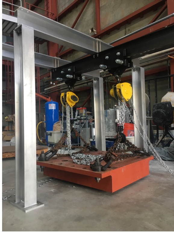
Figure 2.12: Photo of the hoisting structure during a load test performed at UCSD prior to implementation at the observatory site. The block used as the load during this test weighed about 2500 lbs, significantly more than the weight of the receiver. Though it was successful, diagonal members were added to the design following this test to improve rigidity along the axis parallel to the center trolley beam.
