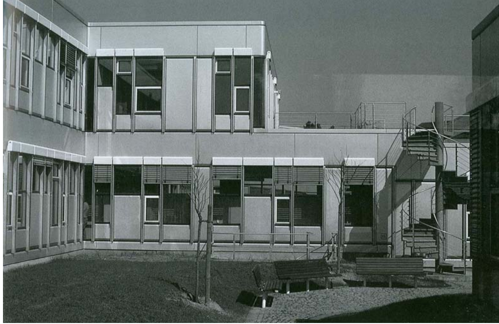
Fig. 14. Spiral staircases in the small courtyards and the Cor-ten covered façade with shading mechanisms. Gabriel Feld, and Peter Smithson. Free University, Berlin : Candilis, Josic, Woods, Schiedhelm. Exemplary Projects, 3 (London: Architectural Association, 1999; 77).
