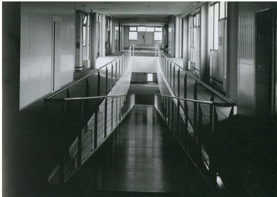
Fig. 13. Ramp within the primary Stem. Gabriel Feld, and Peter Smithson. Free University, Berlin : Candilis, Josic, Woods, Schiedhelm. Exemplary Projects, 3 (London: Architectural Association, 1999; 83).
