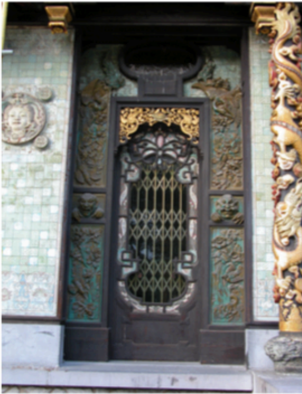
Figure 41. Section of lower façade, the Chinese Pavilion.
