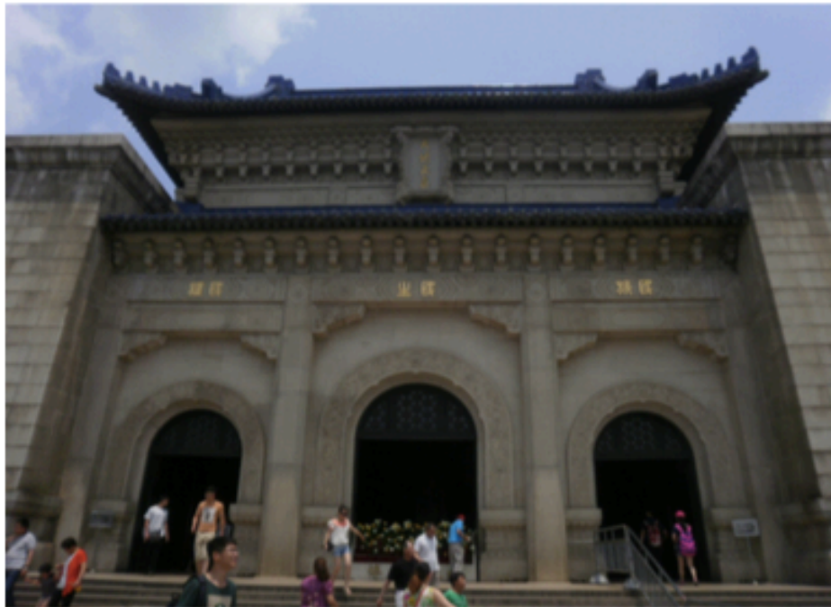
Figure 27. Entrance to the main structure to the Sun Yat-sen Mausoleum, Nanjing, 1926-29.
