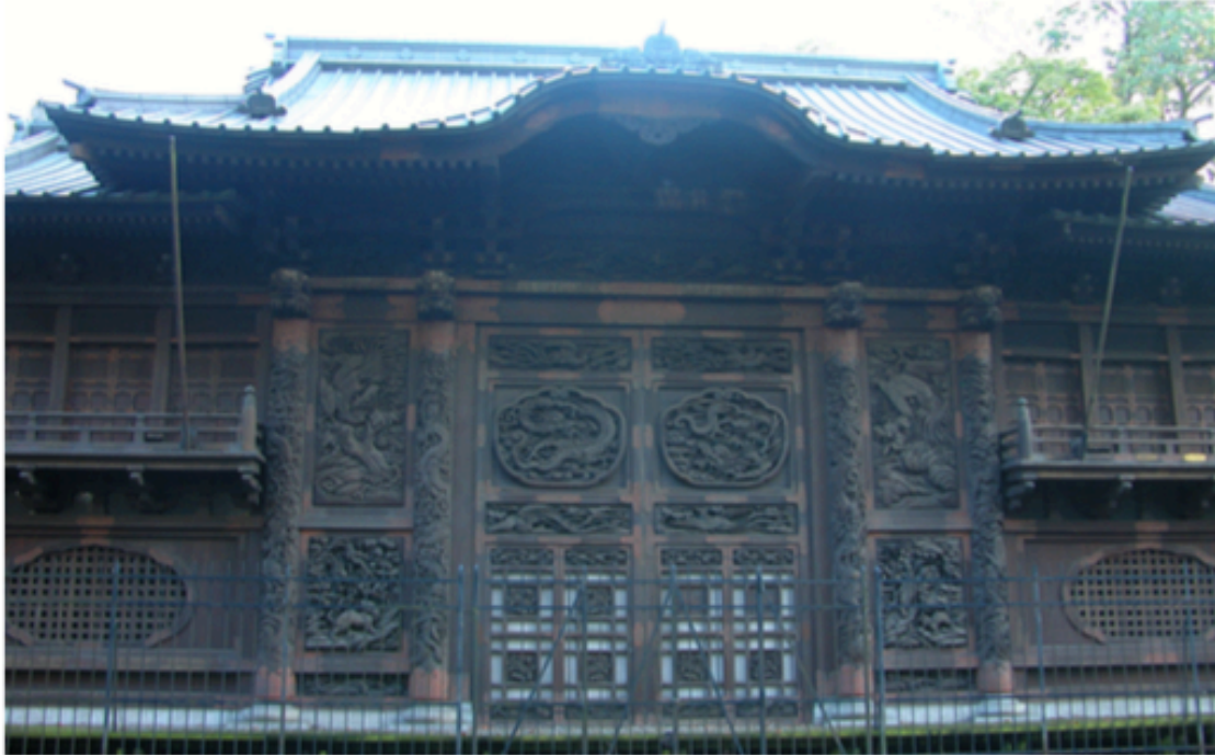
Figure 33. Façade of the annex building for the Japanese Pagoda, Laeken Park, Brussels.
