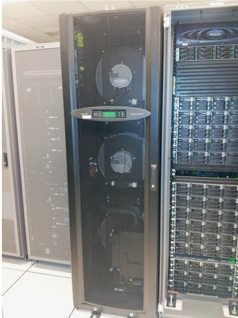
Figure 1-3: Prototype InRow™ Cooling Unit Installed at Lawrence Berkeley National Laboratory for the Demonstration
