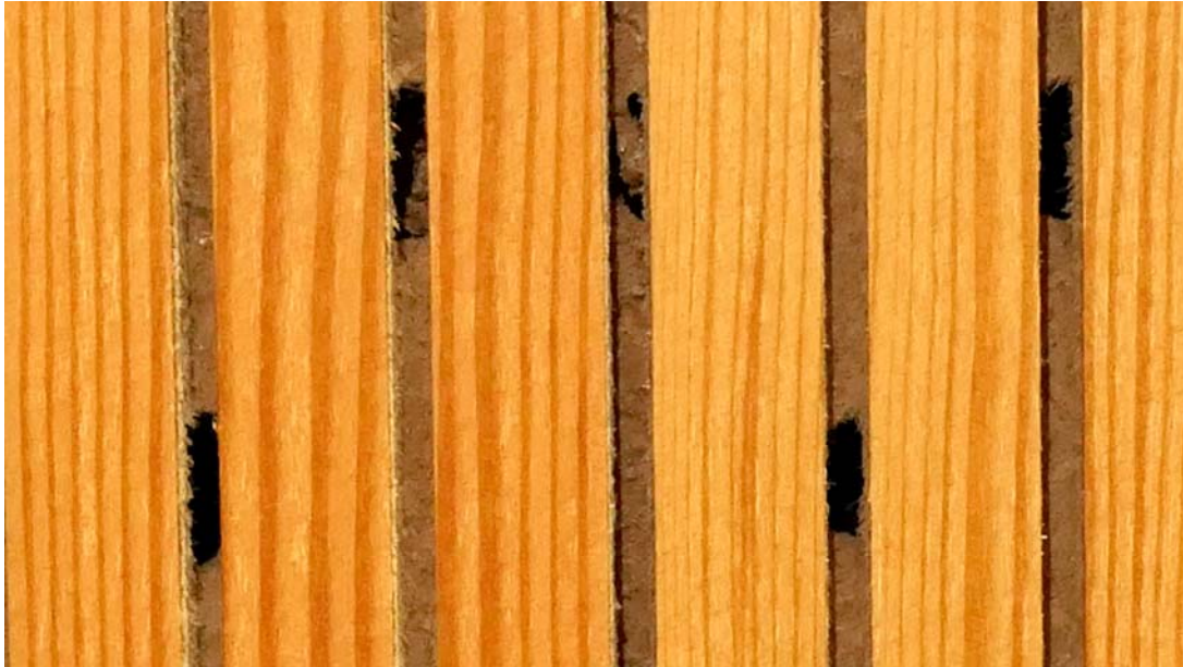
Figure 8: Perforated ACGI Encore I panel (west wall). The dark elongated slots within the grooves are the acoustical perforations that enable sound to “see” the absorptive material behind the wood surface Photo Credit: Charles Salter (edited by Chelsea Hall)
