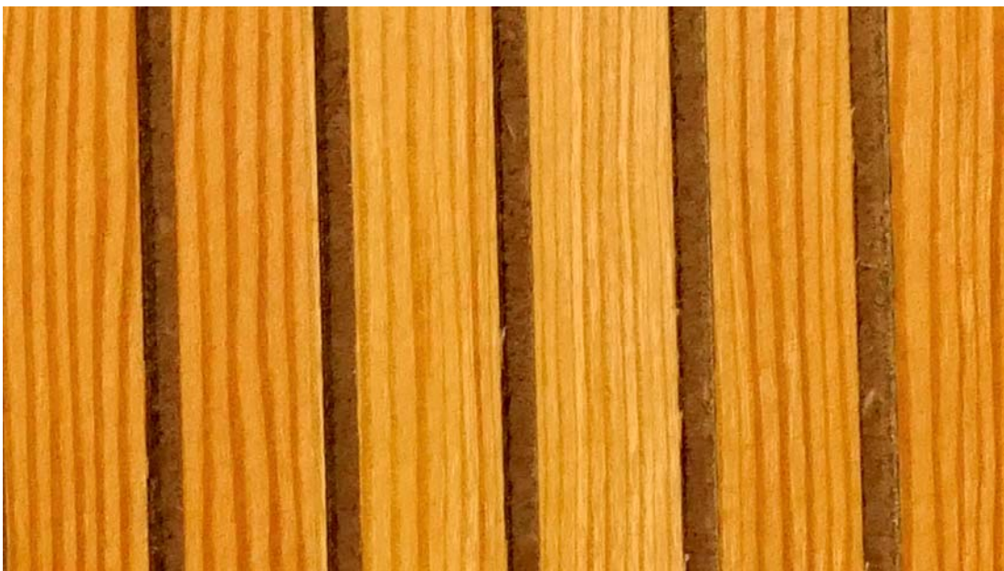
Figure 9: Non-perforated ACGI Encore I panel (east wall) Photo Credit: Charles Salter
