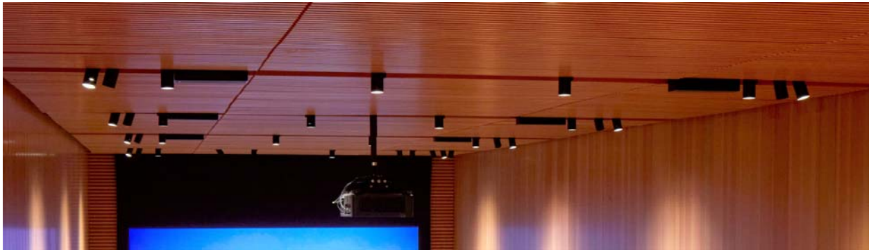
Figure 14: Loudspeakers recessed in ceiling of lecture hall (view from rear) Photo Credit: Richard Barnes (edited by Chelsea Hall)
