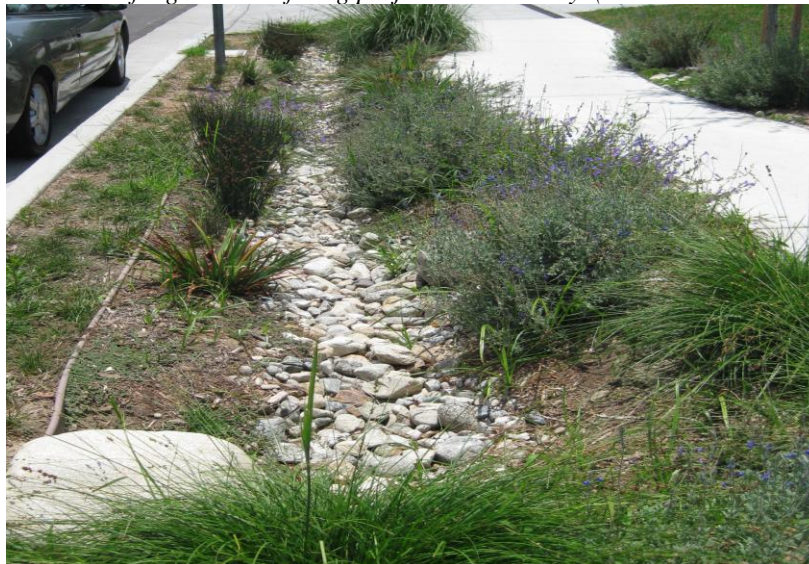
Figure 3.3. Bioswales of a green retrofitting project in Sun Valley. (Source: Photo taken by author.)
