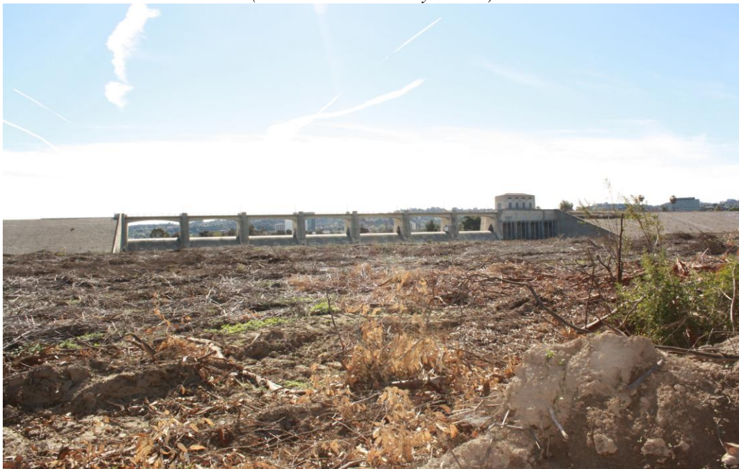
Figure 1. The Sepulveda Basin after bulldozing by the Army Corps of Engineers. (Source: Photo taken by author.)
