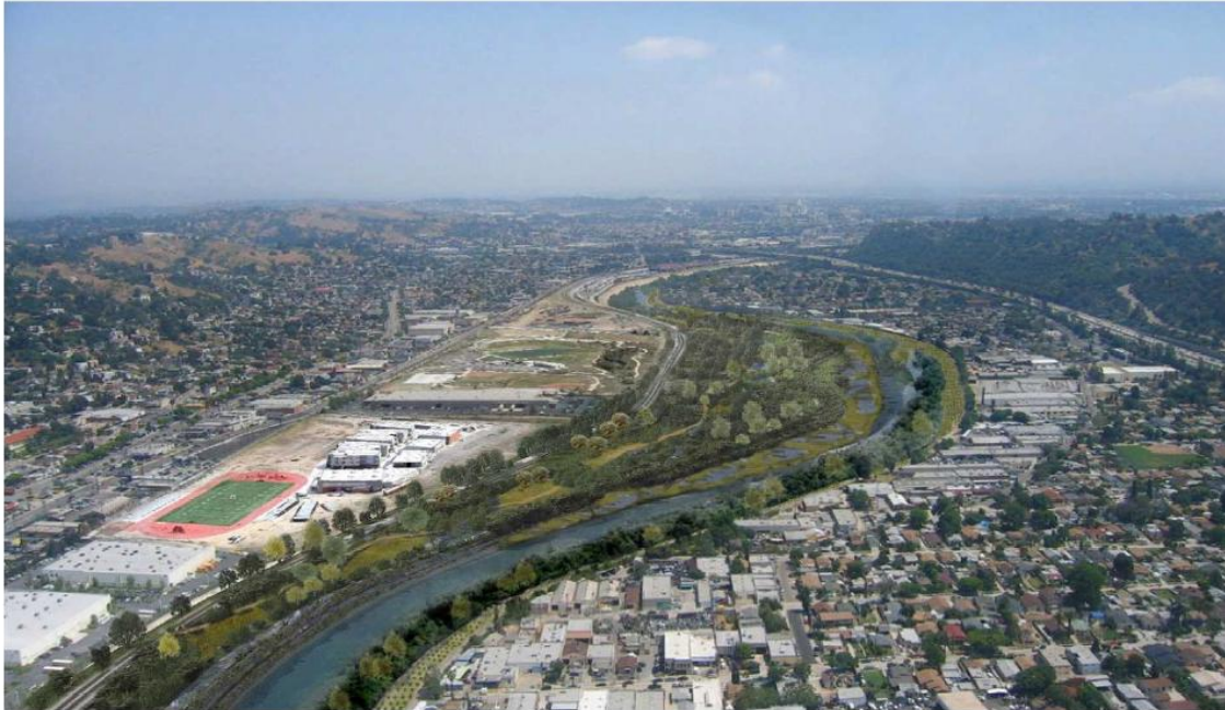
Figure 4.1. A rendering of parks and wetlands at the Taylor Yards after river restoration. (Source: U.S. Army Corps of Engineers 2013 ARBOR Study.)
