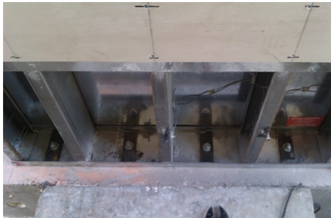
Figure 6.54: Test SSRE010-05 Lower Connection
