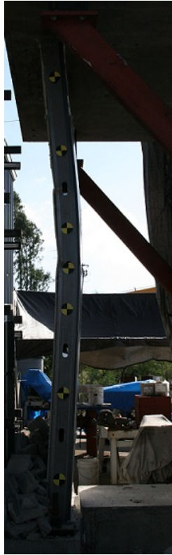
Figure 6.58: Test SSRE010-05 Primary Damage
