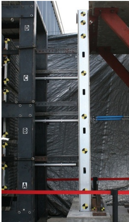
Figure 6.17: Test SSRE010-01 Initial Setup
