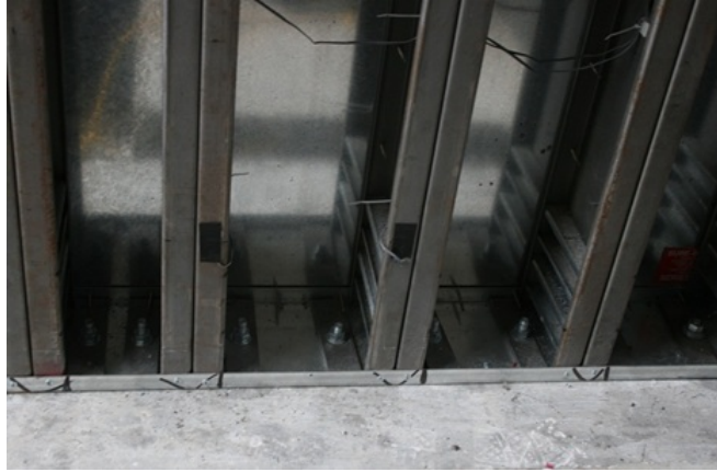
Figure 6.24: Test SSRE010-02.1 Lower Connection
