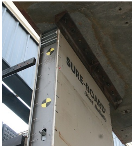
Figure 6.35: Test SSRE010-03.1 Upper Connection
