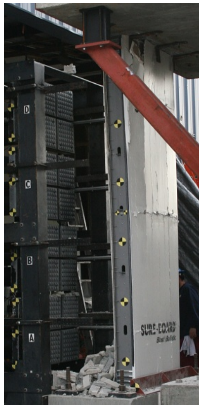
Figure 6.64: Test SSRE010-06 Primary Damage
