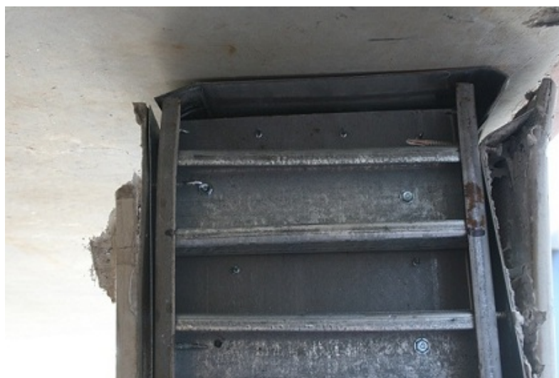
Figure 6.32: Test SSRE010-02.2 Primary Damage
