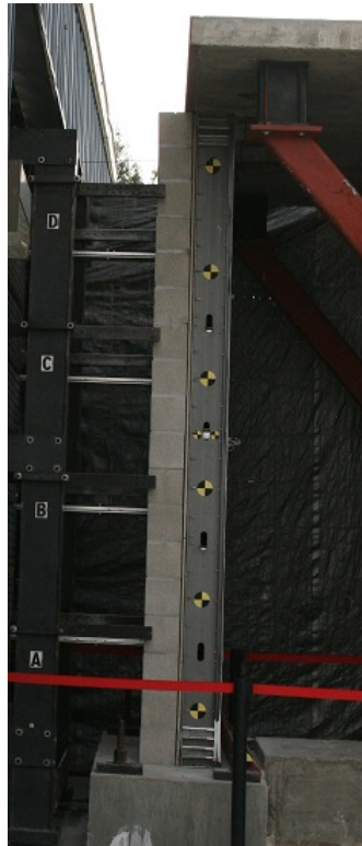
Figure 6.59: Test SSRE010-06 Initial Setup
