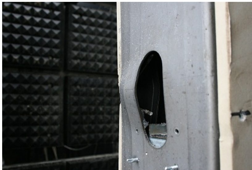
Figure 6.51: Test SSRE010-04.1 Primary Damage
