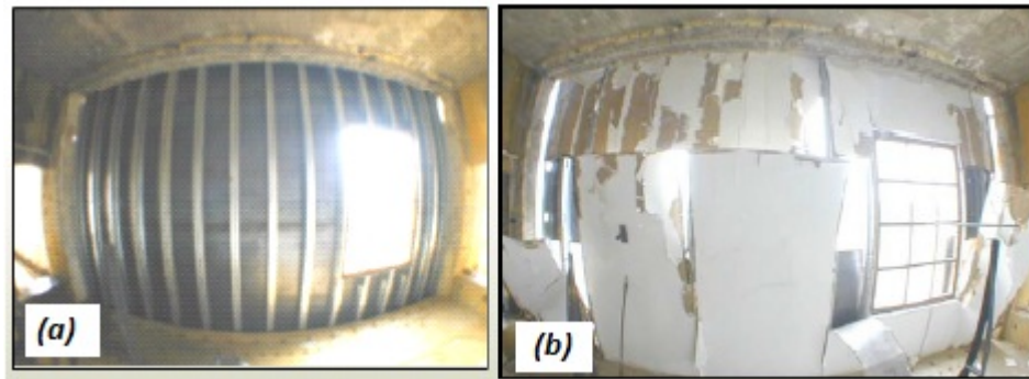
Figure 6.1: (a) Studs prior to blast (b) interior view after blast [50]
