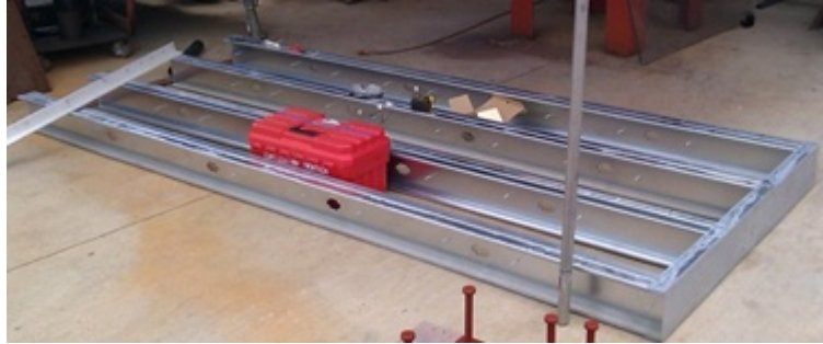
Figure 6.7: Preliminary stud-track assembly
