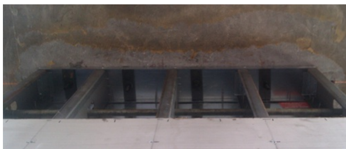
Figure 6.55: Test SSRE010-05 Upper Connection
