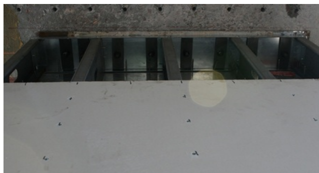
Figure 6.46: Test SSRE010-04.1 Upper Connection
