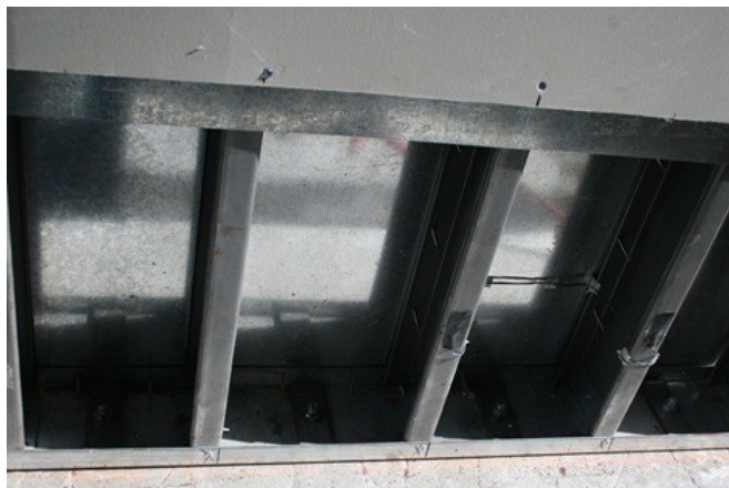
Figure 6.45: Test SSRE010-04.1 Lower Connection
