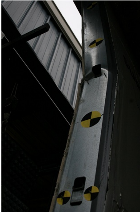
Figure 6.70: Test SSRE010-07 Primary Damage
