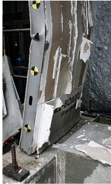
Figure 6.52: Test SSRE010-04.2 Damage
