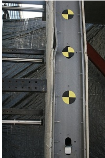
Figure 6.42: Test SSRE010-03.2 Primary Damage
