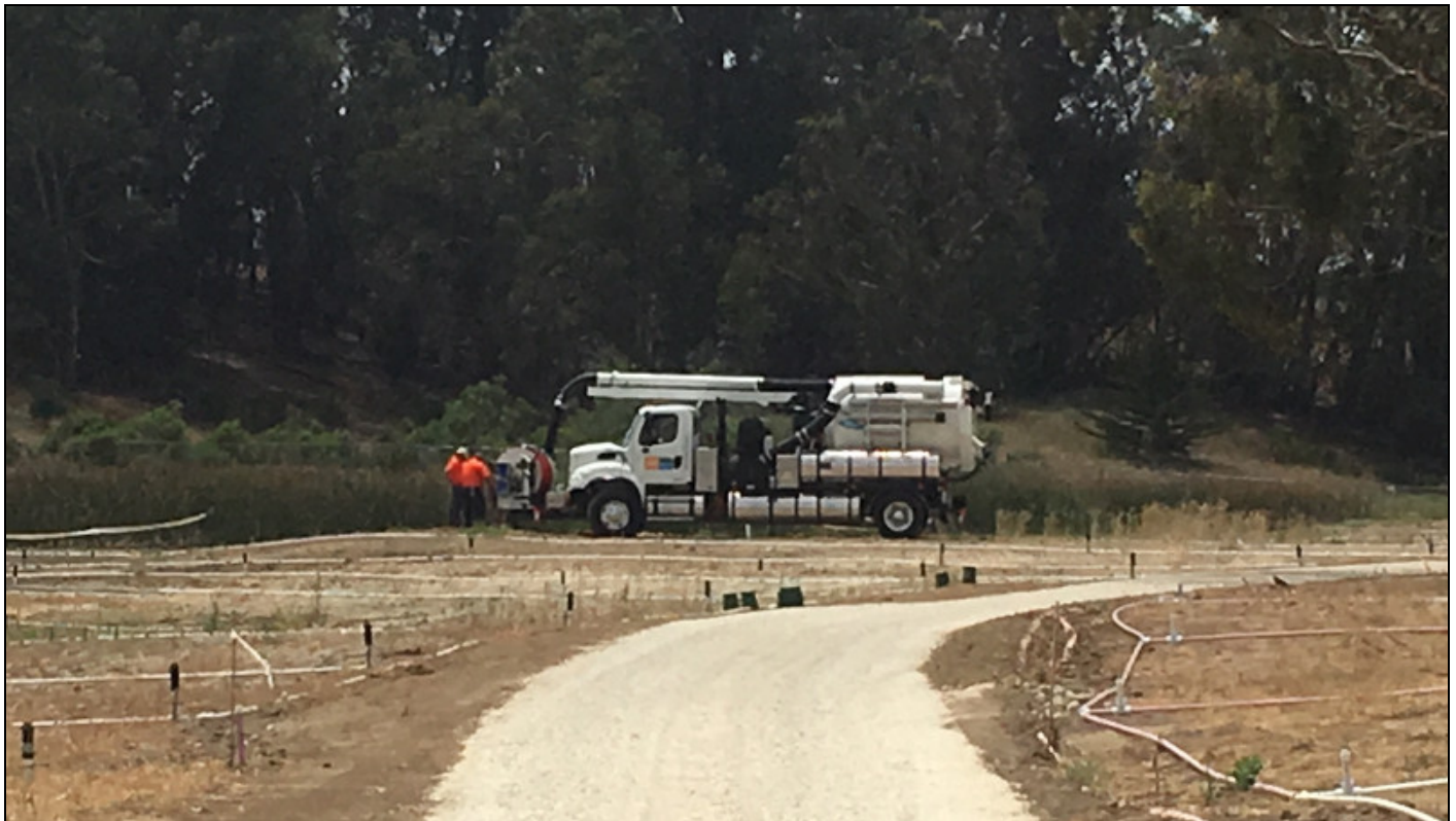
A Goleta West Sanitary District maintenance vehicle accessing a sewer line manhole in the western arm of NCOS.
