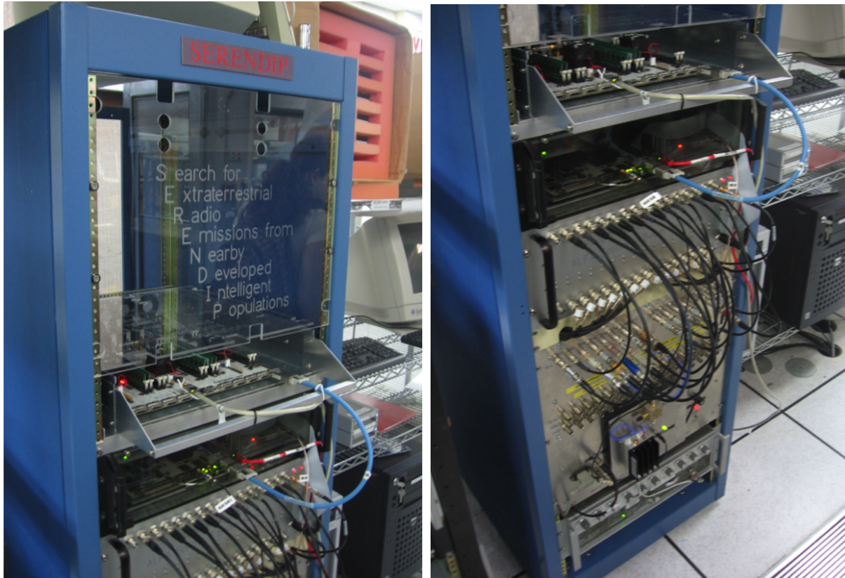
Figure 3.11: SERENDIP V.v Hardware installed at Arecibo Observatory
