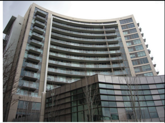
Residential Tower, Hoyt Street Properties, Portland
