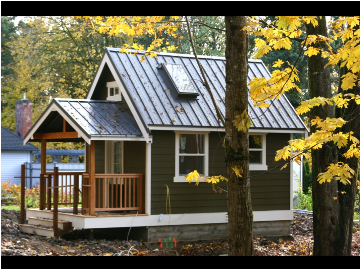
Figure 49: Photograph of a small Accessory Dwelling Unit (ADU). Courtesy of New Avenue Homes.
