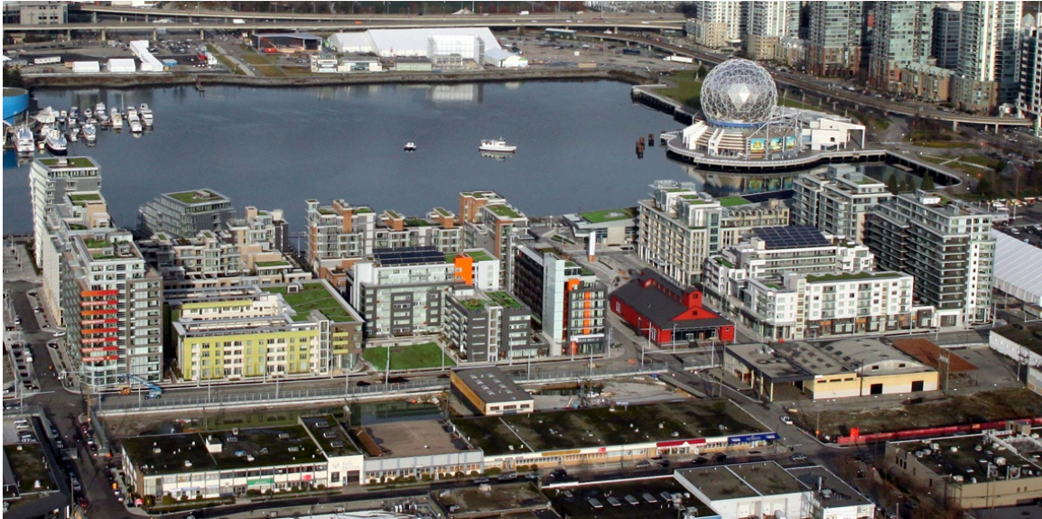
Figure 15: Aerial of SE False Creek, courtesy of Scot Hein, City of Vancouver (2011)
