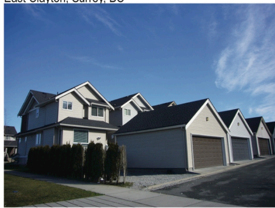
Single-family units with coach houses, East Clayton
