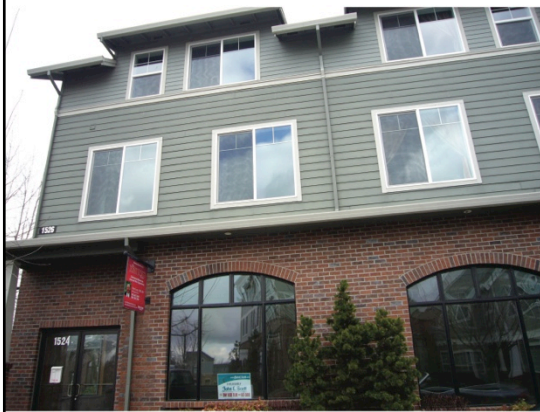
Commercial below, residential above (Live-work units, Fairview Village, OR
