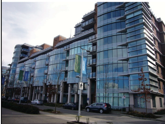
Multi-Unit Apartment building, Southeast False Creek
