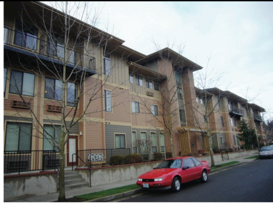
Apartment Building, Fairview Village, OR
