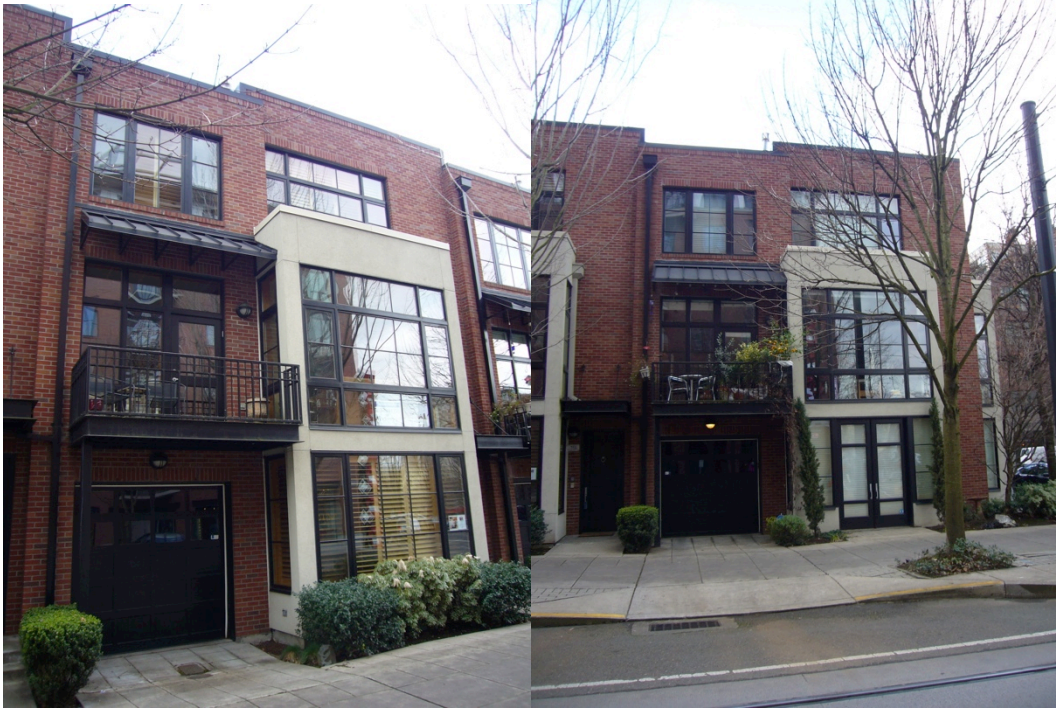
Figure 21: Johnson Street Townhomes in Pearl District, designed by Mithun Architects (Szibbo 2013)
