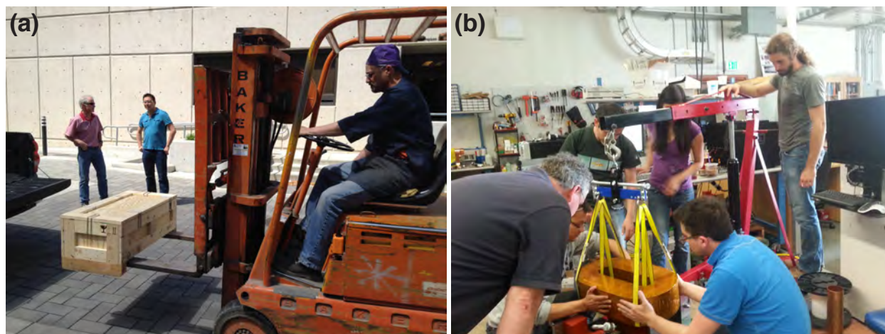
Figure 3.23: Coil Transportation & Assembly. (a) A forklift was used to move each coil onto a steel dolly for transportation. (b) The coils were lowered onto the iron return assembly and centered using an engine hoist, a load leveler, and web slings.
