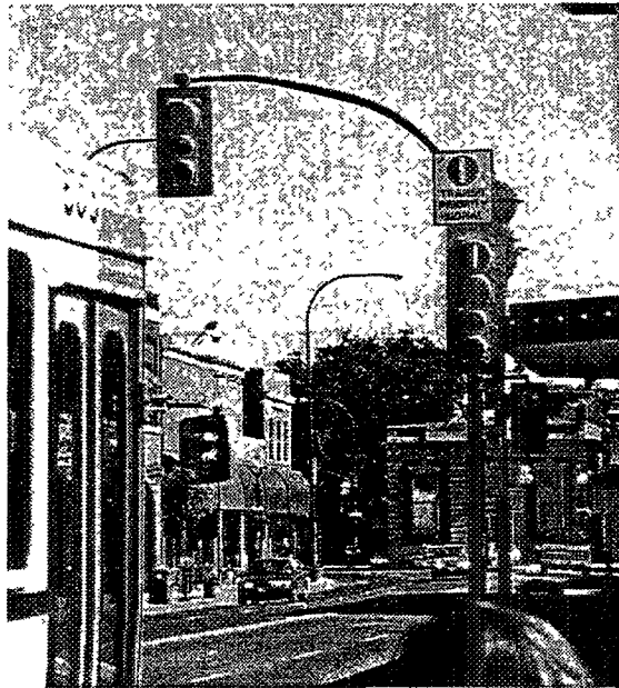
Photo 9.3. A transit priority signal in operation. The vertical white light signals the bus to proceed, while the light stays red for automobiles.
