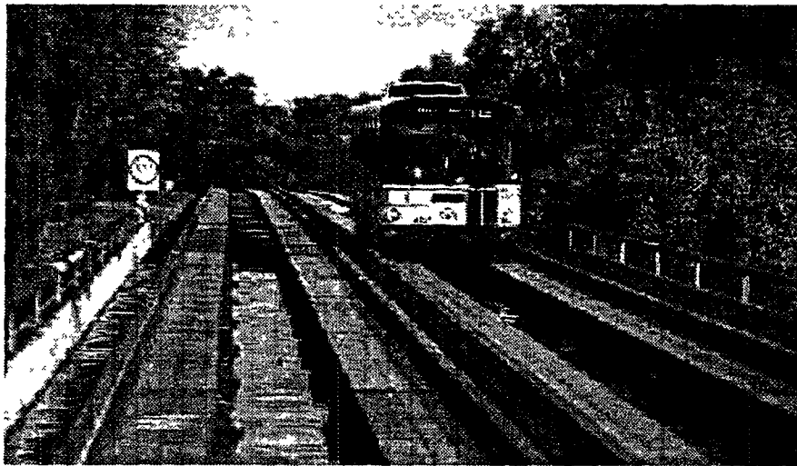
Photo 7.1. Adelaide's Track Guided Busway. A conventional coach equipped with roller guides is steered along a tree-lined busway corridor.
