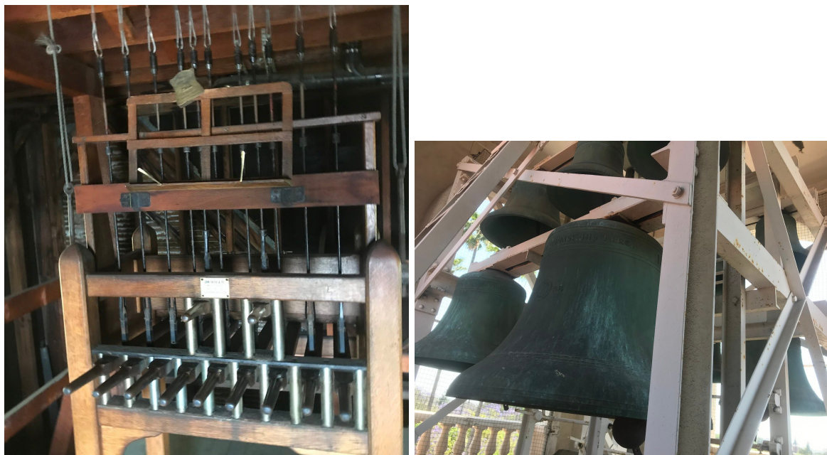
Figs. 2 and 3. Eleven-bell chime leverboard and the bell scaffolding one floor above. 54
