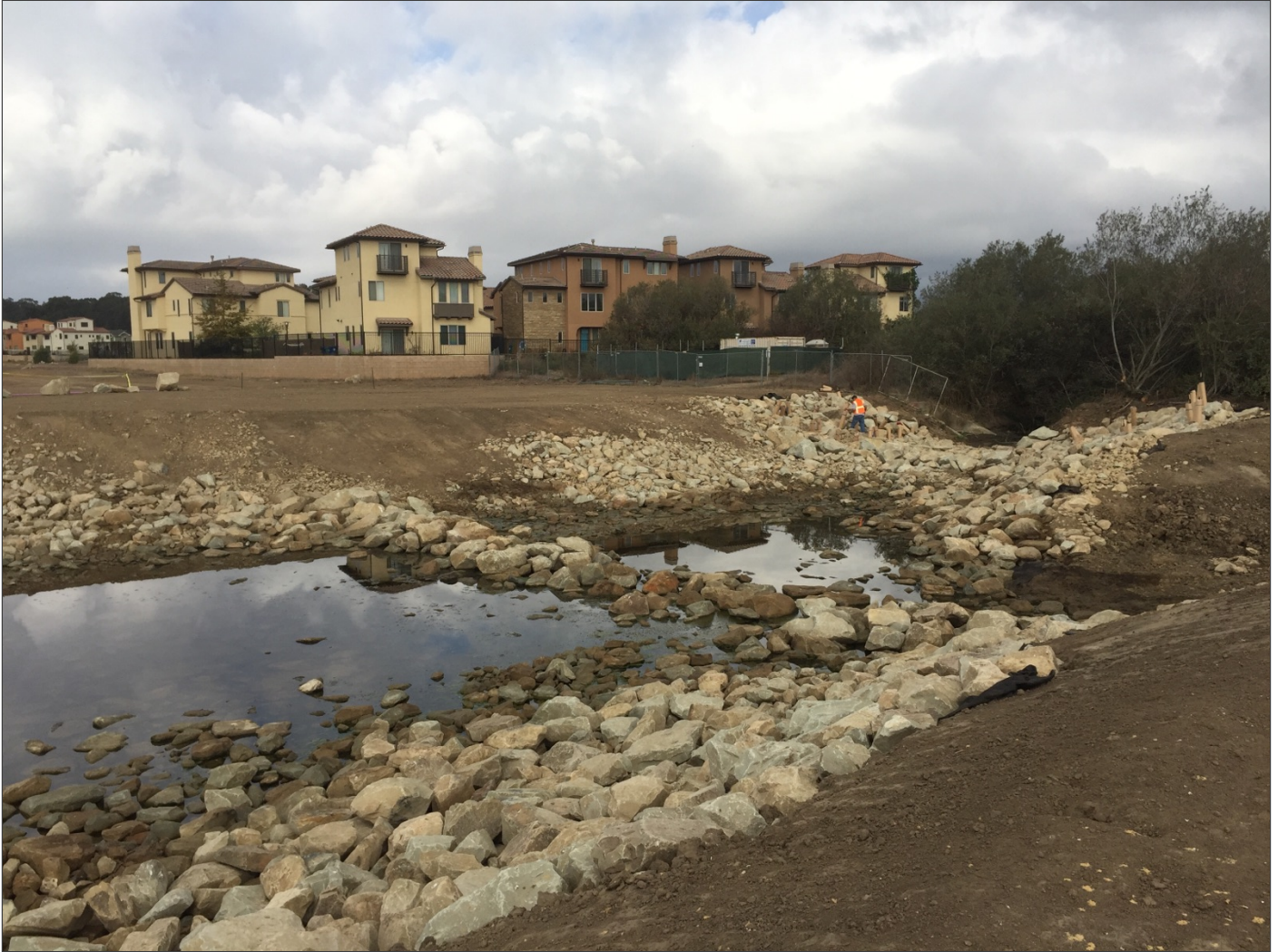
Figure 2. Picture of the boulder lined pools constructed where Phelps Creek enters the NCOS restoration project site.
